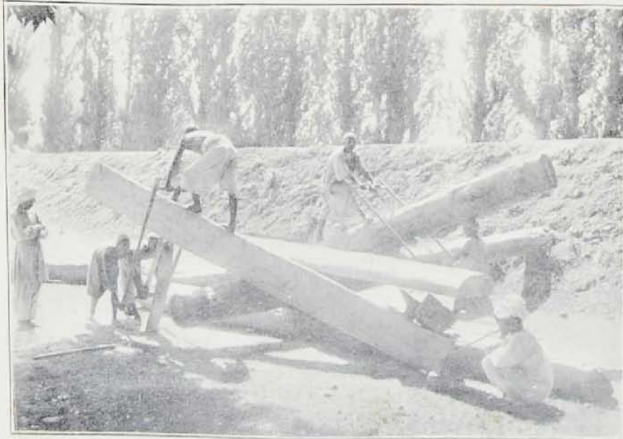
281 WOOD SAWING IN INDIA
