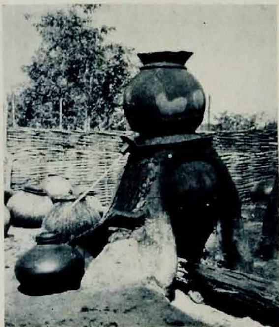
Apparatus for distilling mahua spirit
