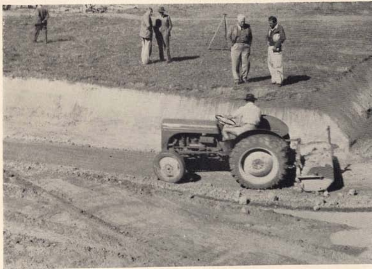
2. Constructing a T-dam in Rhodesia.
