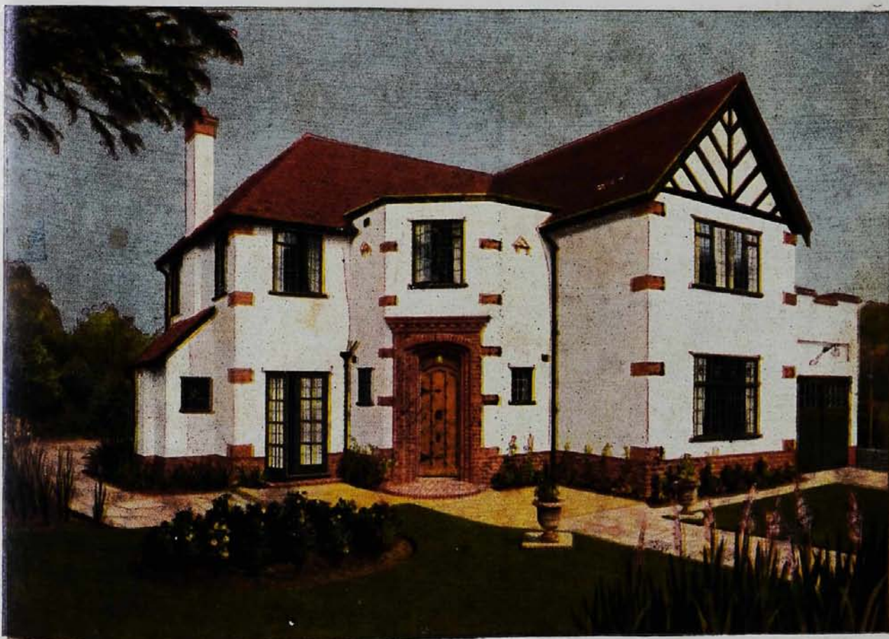
"SNOWCRETE" AND "COLOCRETE" FOR DOMESTIC ARCHITECTURE. House faced with "Snowcrete". Roof of concrete tiles. Approach and garden paths of coloured Portland cement concrete resembling natural stones.
