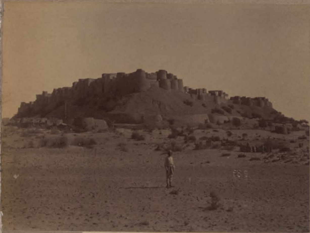
Jesulmir Fort from the South-West.
