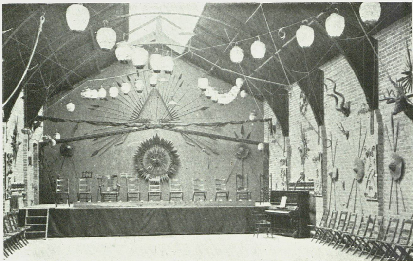
INTERIOR OF GYMNASIUM AND ASSEMBLY ROOM
