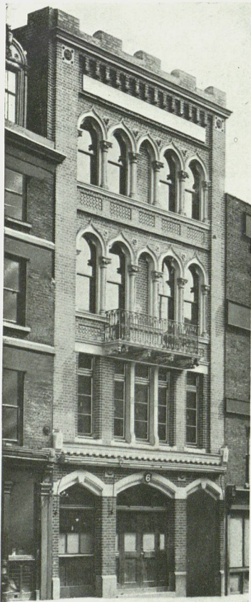
WELLCOME CHEMICAL RESEARCH LABORATORIES KING STREET, LONDON (ENGLAND)
