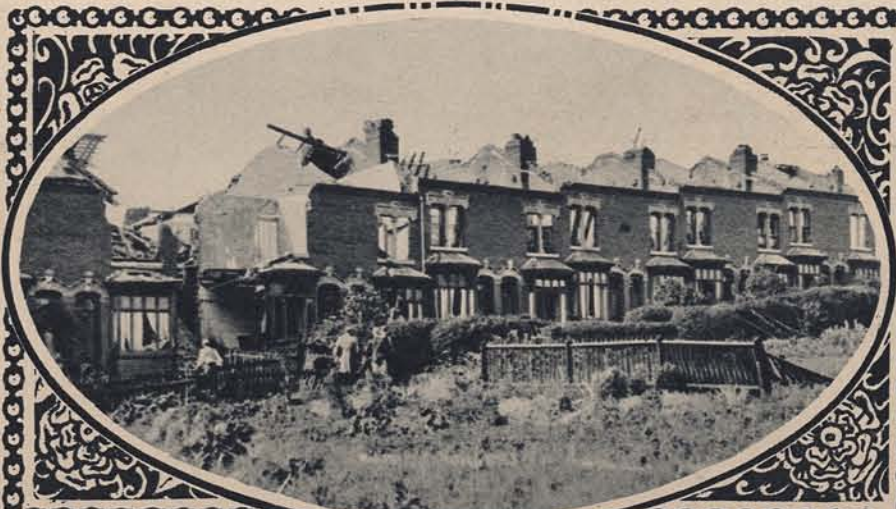
1931: A CYCLONIC GALE AT BIRMINGHAM—A WHOLE ROW OF HOUSES IN FORMAN'S ROAD, SPARKHILL, WITH THEIR ROOFS RIPPED OFF. An almost unique event in the varied records of English weather was the windstorm which devastated parts of Birmingham on June 14, 1931. It was described as a small tropical tornado or cyclone. It pursued a track about half a mile wide and eight miles long through the eastern side of the city, leaving a clearly defined belt of destruction. One woman was killed by the collapse of a wall in Forman's Road.
