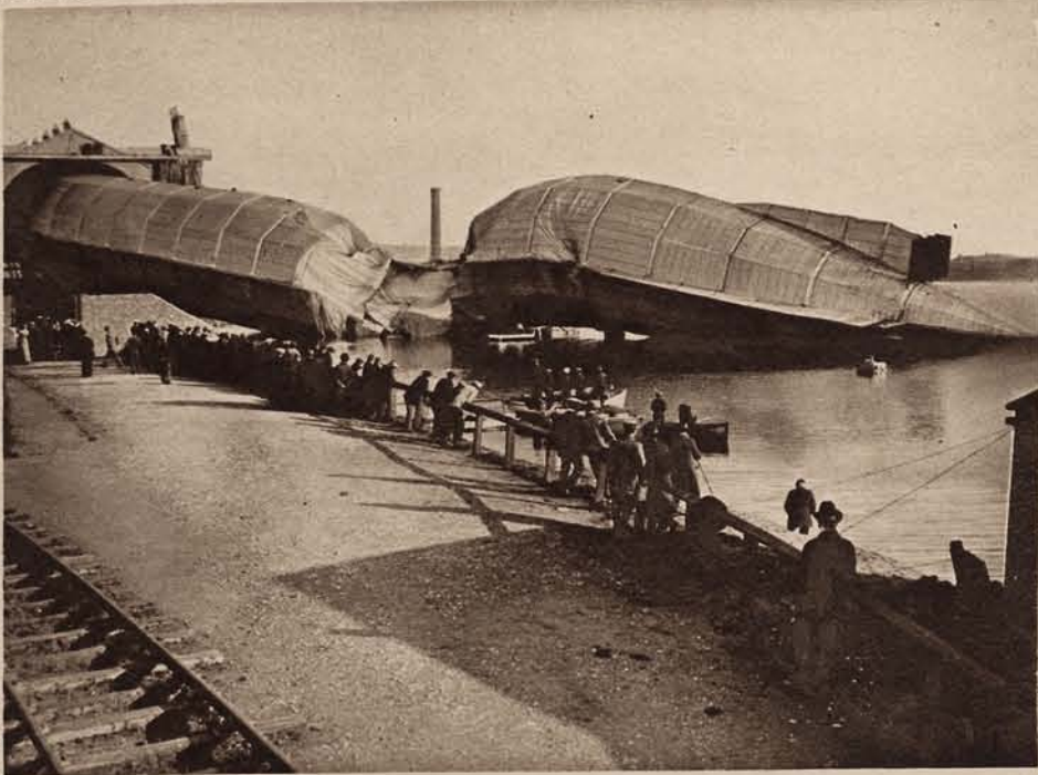
1911: THE FIRST BRITISH RIGID AIRSHIP BREAKS HER BACK BEFORE EVER FLYING—THE "MAYFLY" WRECKED ON COMING OUT FOR HER FIRST TRIAL. The series of misfortunes which have throughout dogged the British airship industry began on September 23, 1911, when the naval dirigible "Mayfly," built at Barrow for the Admiralty by Messrs. Vickers at a cost of £40,000, was wrecked when being taken out of her shed for her first trial. The airship was caught by the wind, heeled over, and eventually broke her back. No lives were lost in the disaster.
