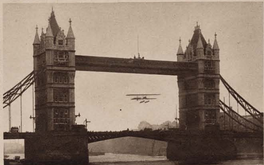
1912: FLYING BETWEEN THE UPPER AND LOWER SPANS OF THE TOWER BRIDGE—A HAZARDOUS FEAT BY MR. F. K. MCCLEAN. In August 1912, Mr. F. K. McClean, on a business visit to London, decided to fly from Eastchurch in his Short seaplane. He followed the course of the Thames, and not only passed between the upper and lower spans of the Tower Bridge, but flew underneath all the four remaining bridges to Westminster, where he alighted. The police made him taxi all the way back to Shadwell Basin.
