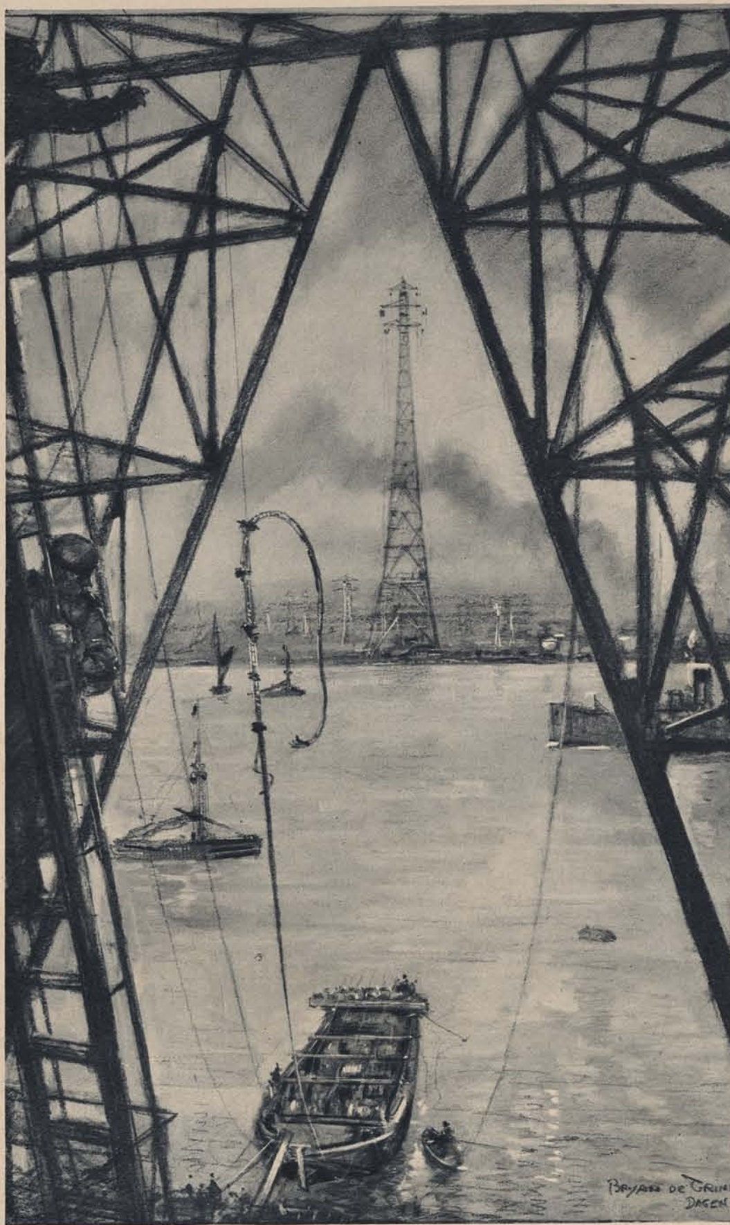
1927: THE GRID—THE "ELECTRIFICATION" OF BRITAIN BY MEANS OF A CONNECTED SYSTEM OF "PYLONS": CARRYING CONDUCTORS ACROSS THE THAMES FROM DAGENHAM TO KENT.
