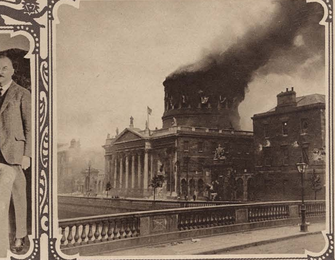
1922: THE DOME OF THE FOUR COURTS ABLAZE DURING FIGHTING IN DUBLIN BETWEEN FREE STATE TROOPS AND REPUBLICAN REBELS. Severe fighting took place in Dublin in June and July 1922, between troops of the Irish Free State Government and Republicans. The Four Courts, one of the city's finest buildings, was sacrificed, as the Republicans had made it their headquarters. Bombardment set it on fire, and it was surrendered on June 30. Thereafter the rebels held out for some days in a group of fortified hotels.
