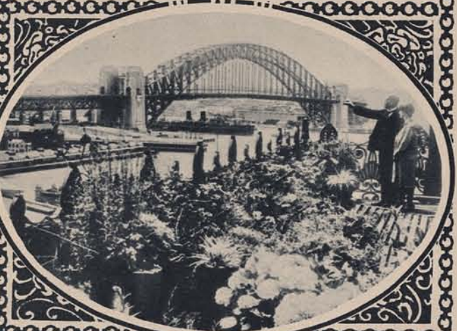
1932: THE SYDNEY HARBOUR BRIDGE—ONE OF THE GREATEST OF MODERN ENGINEERING FEATS. The Sydney Harbour Bridge, the greatest bridge in the world, was formally opened on March 19, 1932. It spans the harbour between Dawes Point and Milson Point. Its total length is 3770 feet, and ships taller than the Nelson column can pass below the main span at high tide.
