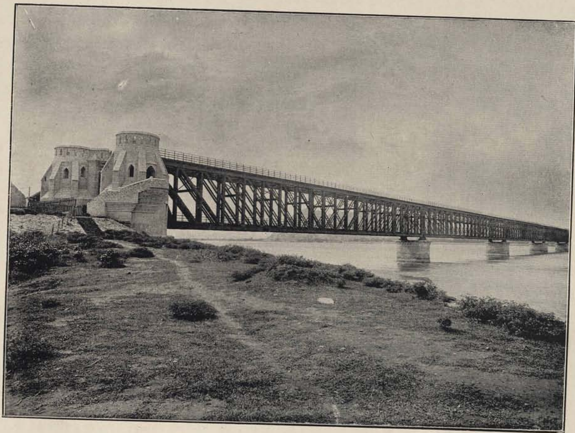
BRIDGE OVER THE KISTNA RIVER—BEZWADA.
