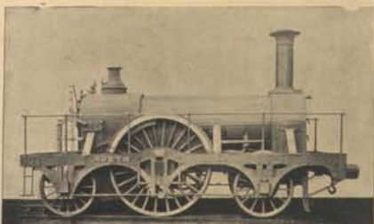
GREAT WESTERN RAILWAY BROAD-GAUGE ENGINE, "NORTH STAR" Built 1827. Run until 1859
