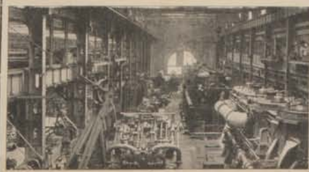
THE GROWTH OF BRITISH SHIPBUILDING The view represents the master engines in the building shop at Clydebank, which covers an area of 72 acres
