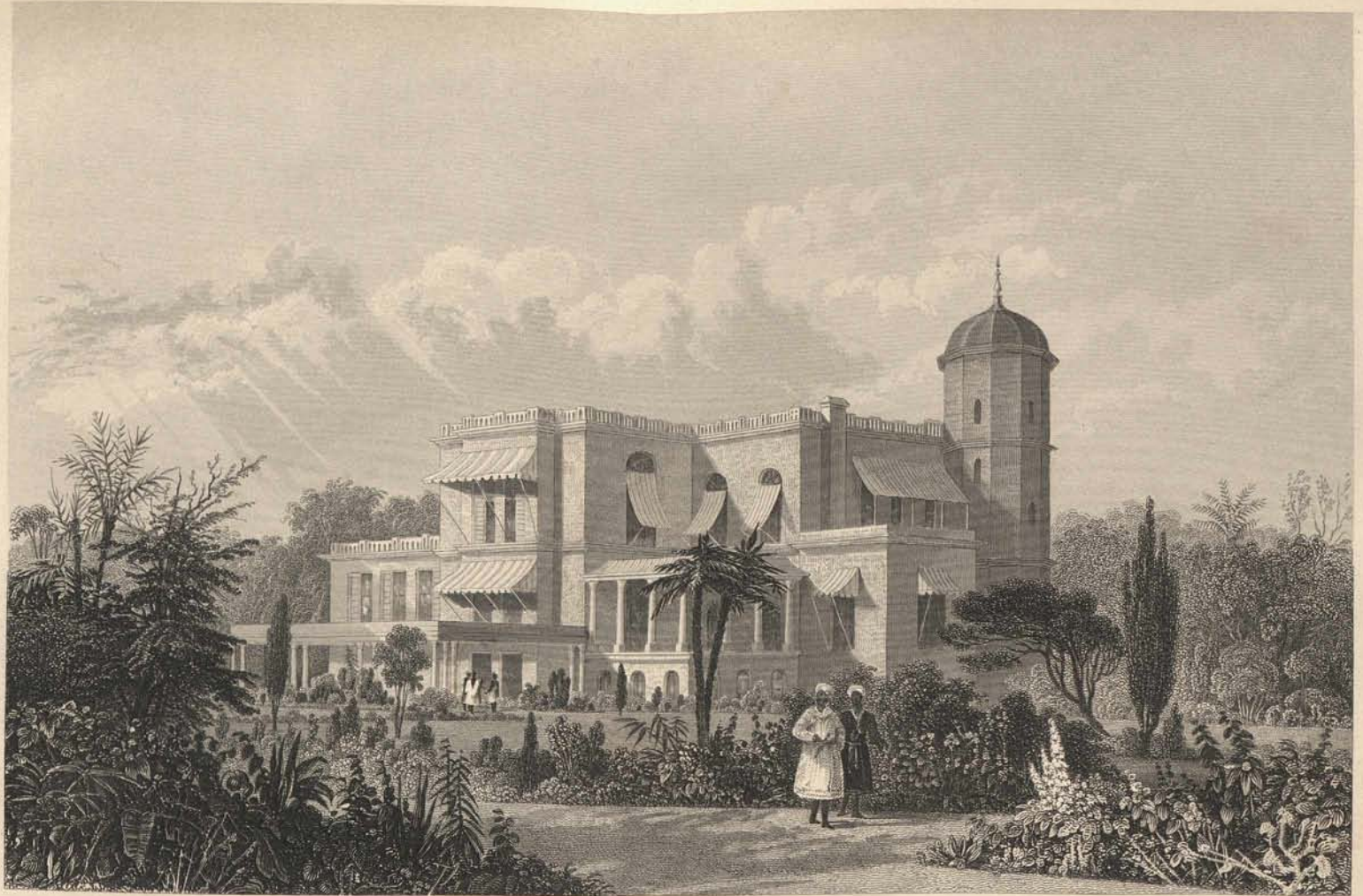
THE RESIDENCY, LUCKNOW.
