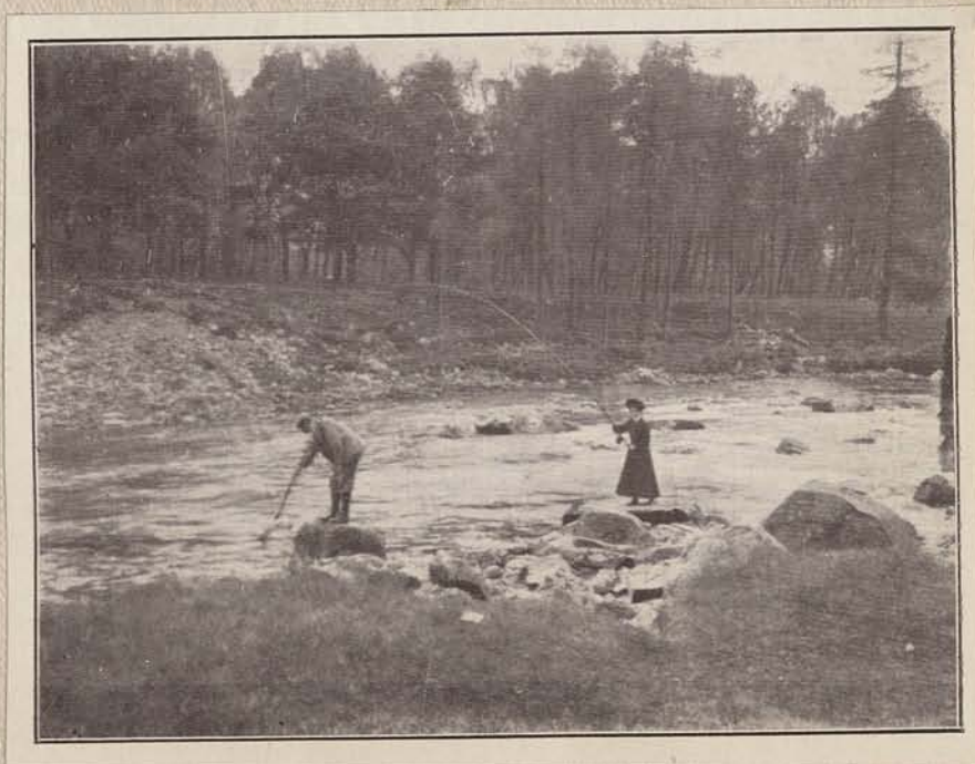
On the Dee at Invercauld Bridge. The Author doing Ghillie.
