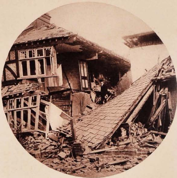
AIR-RAID DAMAGE IN CROYDON
