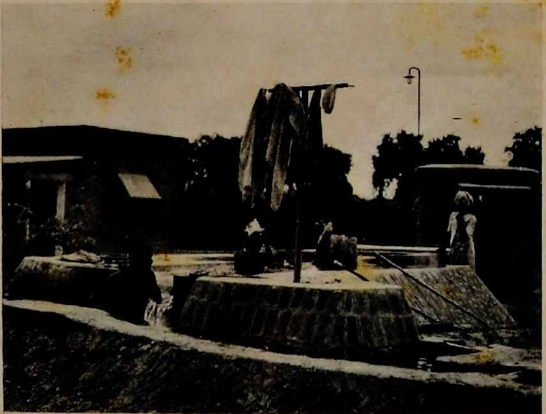
WATER-SUPPLY : NEW STYLE. A TUBE WELL (In Meerut district, United Provinces. This is a State well driven by electricity. The well is in the cylindrical building to the right. In the foreground is a bathing pool. The building to the left is the operator's house. See Chapter I, para. 39.)
