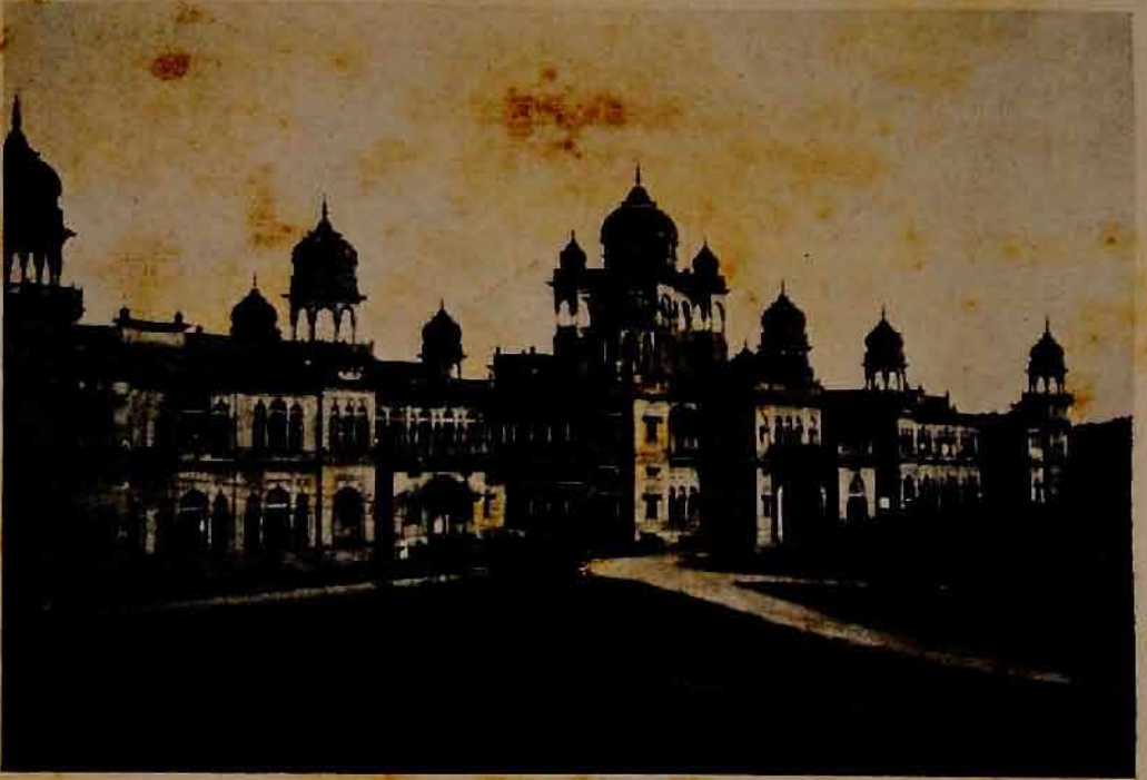
MODERN HOSPITALS King George's Hospital at Lucknow.
