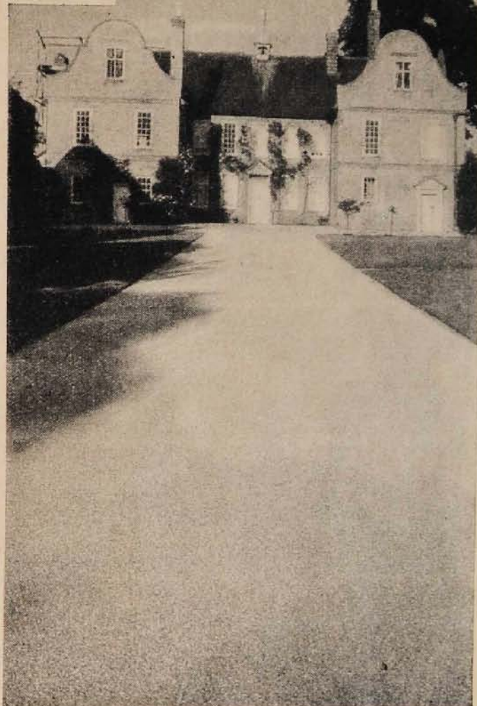
Stoke, Ludlow, Salop. Photo by courtesy of Capt. J. W. D. Evans. Contractors: Grosvenor Workman, Birmingham. Agents for Colas.
