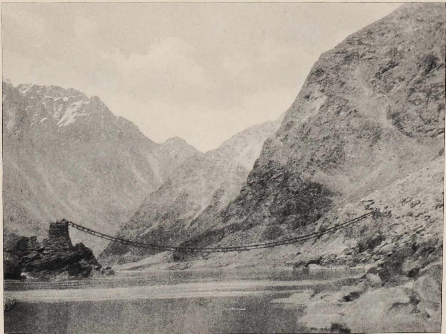
ROPE-BRIDGE AT KARMUNG.
