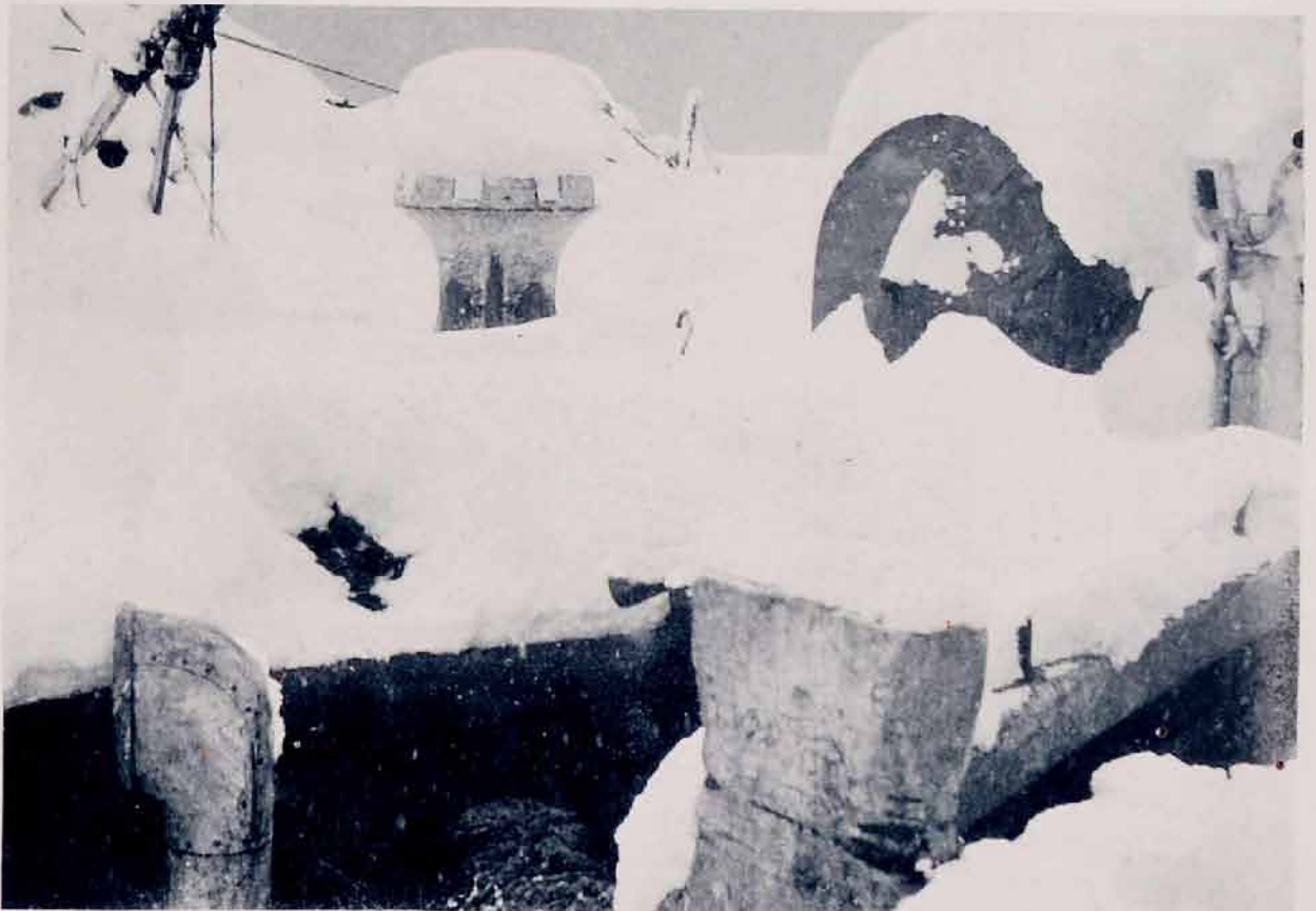
THE DECK OF THE "NIMROD" AFTER A BLIZZARD
