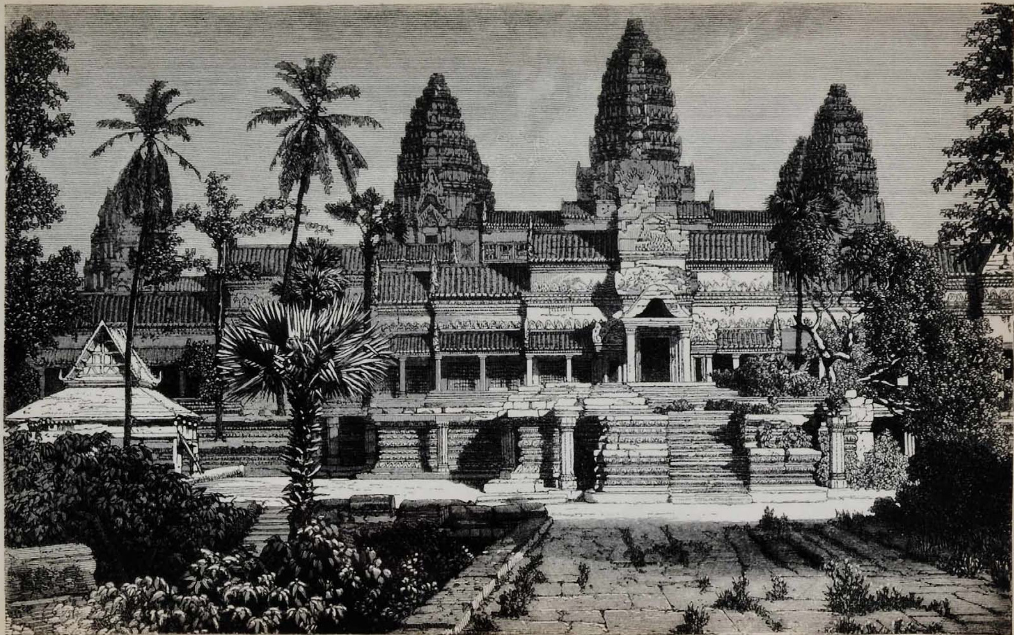
NAGKON WAT: PRINCIPAL FAÇADE
