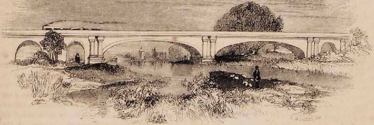
7.—RAILWAY BRIDGE, AND BRAY.
