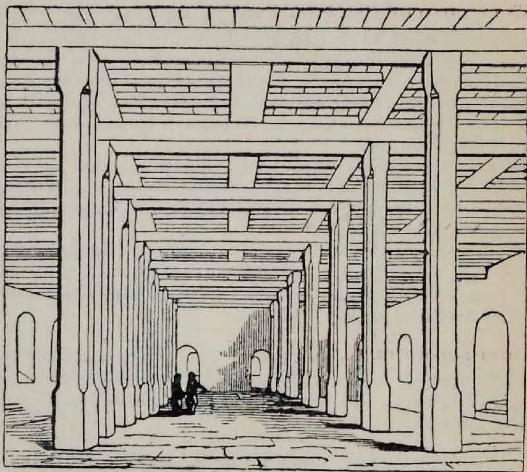
Interior of the Great Council Room on the upper storey of the White Tower. From an engraving by Fairholt.
