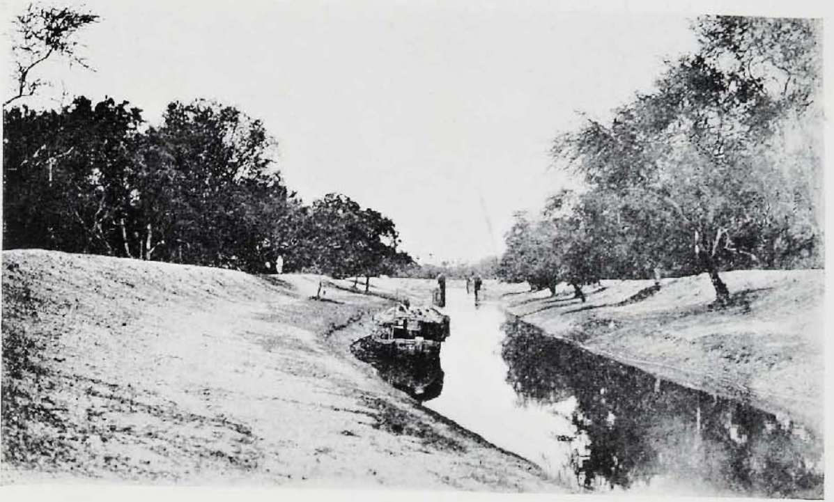
BUCKINGHAM CANAL, NEAR GREENAWAY ROAD, MADRAS
