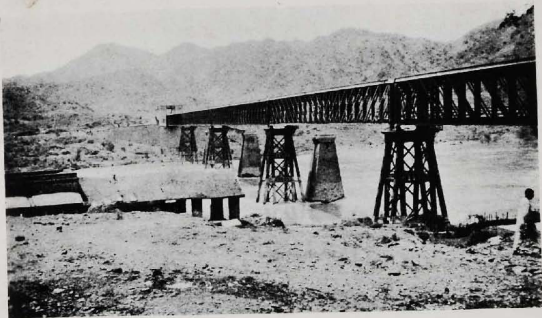
ATTOCK BRIDGE : ACROSS THE INDUS
