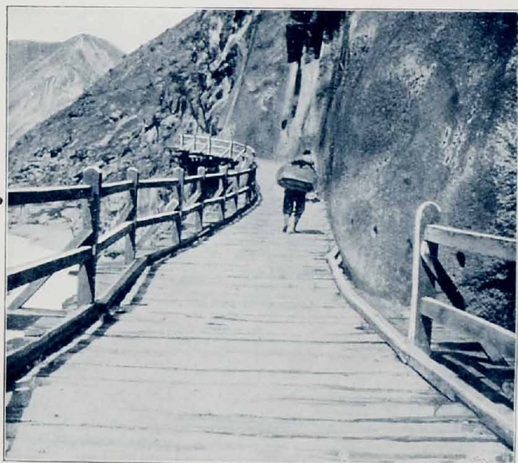
155. THE ROAD IN THE SUTLEJ RAVINE.
