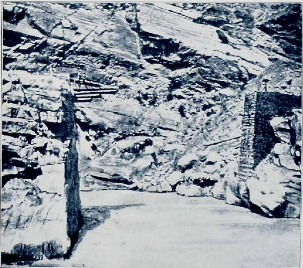
141. WIRE-ROPE BRIDGE NEAR POO.
