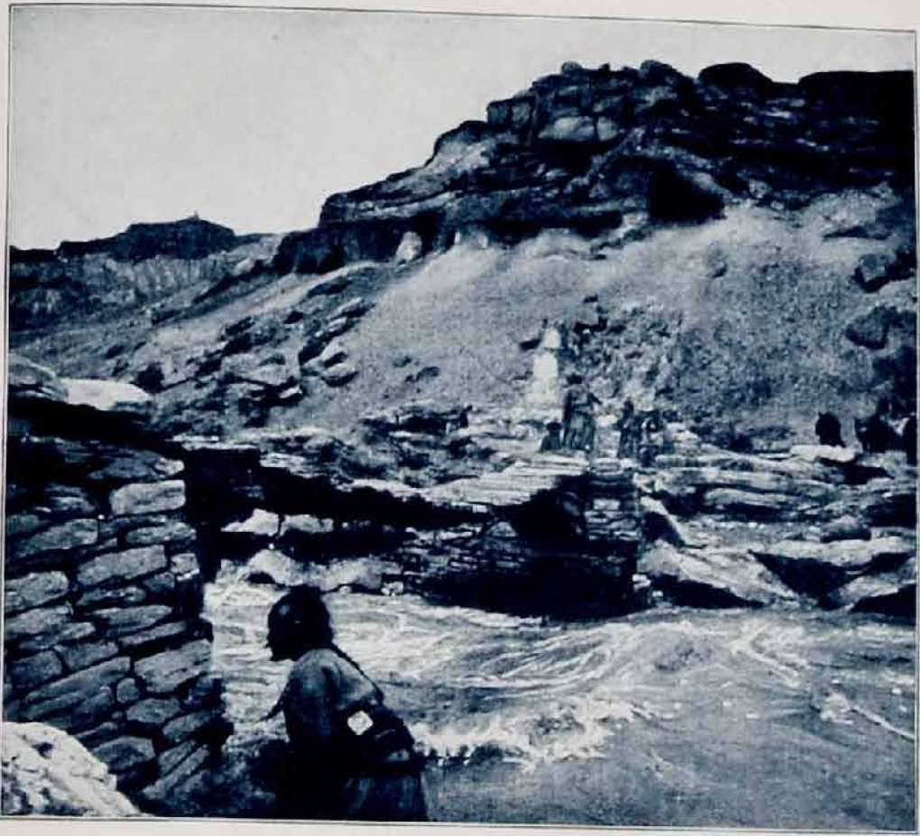
96. THE SUTLEJ BRIDGE NEAR KYUNG-LUNG.
