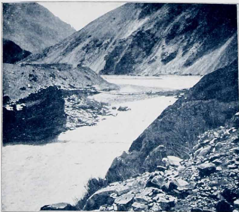
133. THE LOPCHAK BRIDGE.
