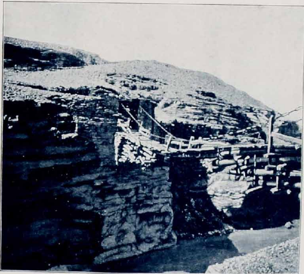
117 AND 118. THE BRIDGE OF TOTLING.
