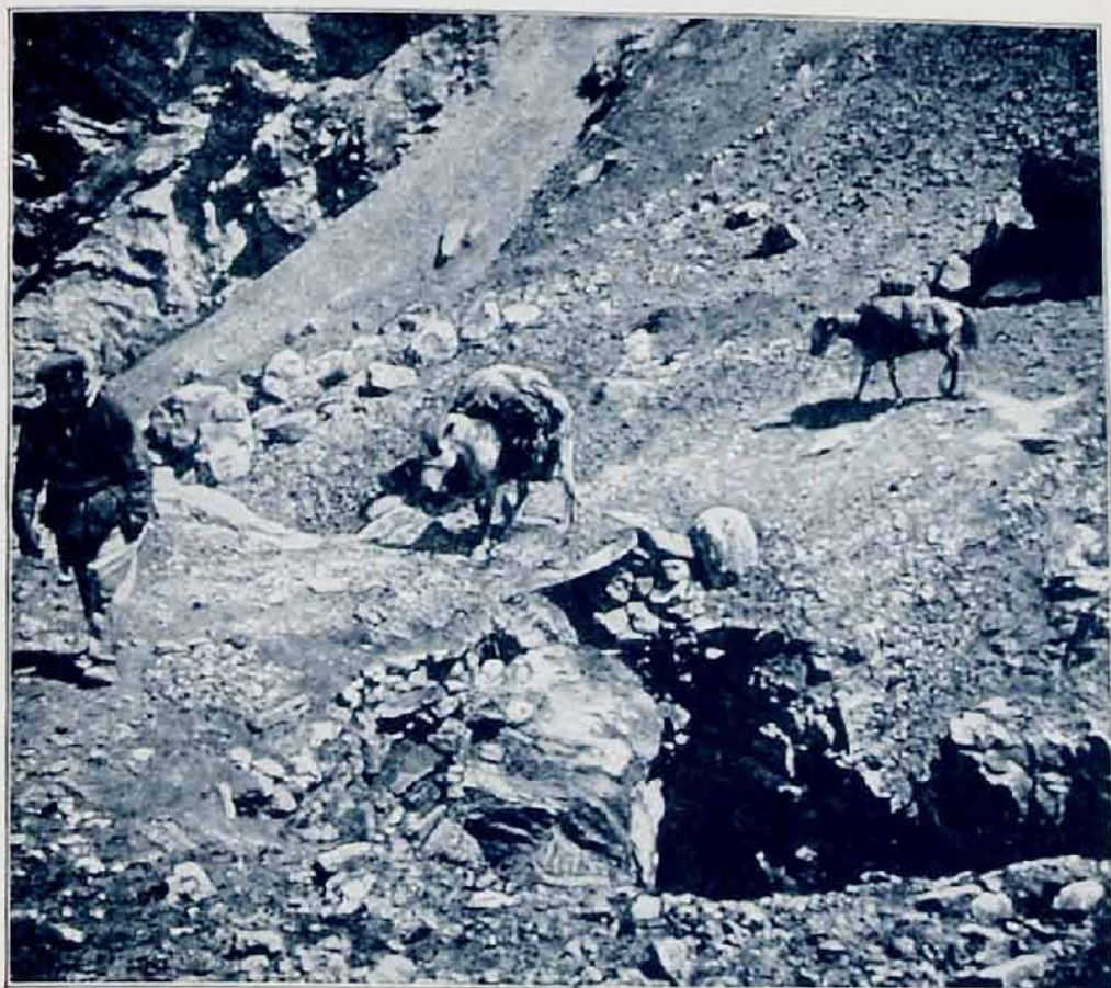
125. THE LITTLE BRIDGE OVER THE NGARI-TSANGPO.
