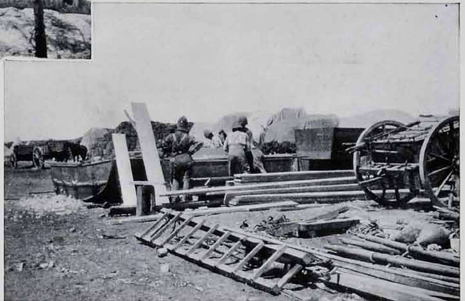
MAKING PONTOONS FOR BRIDGING THE MODDER.
