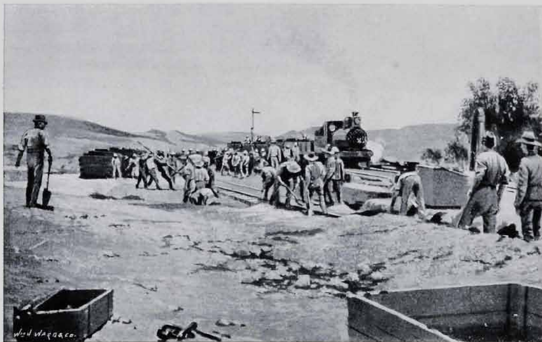
REPAIRING THE RAILWAY NEAR ENSLIN.
