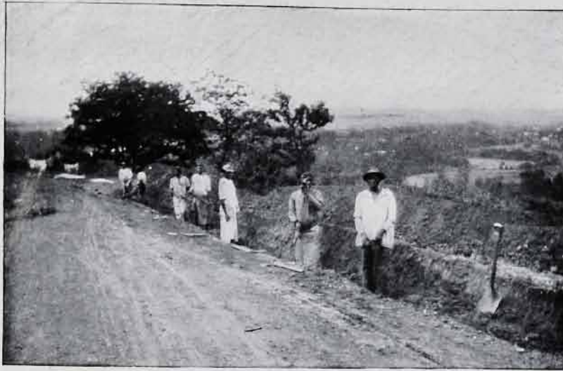
KAFFIRS DIGGING A TRENCH FOR THE BRITISH AT CHIEVELEY.
