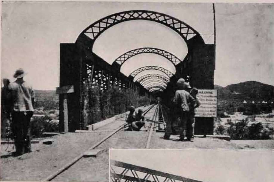
ORANGE RIVER BRIDGE.
