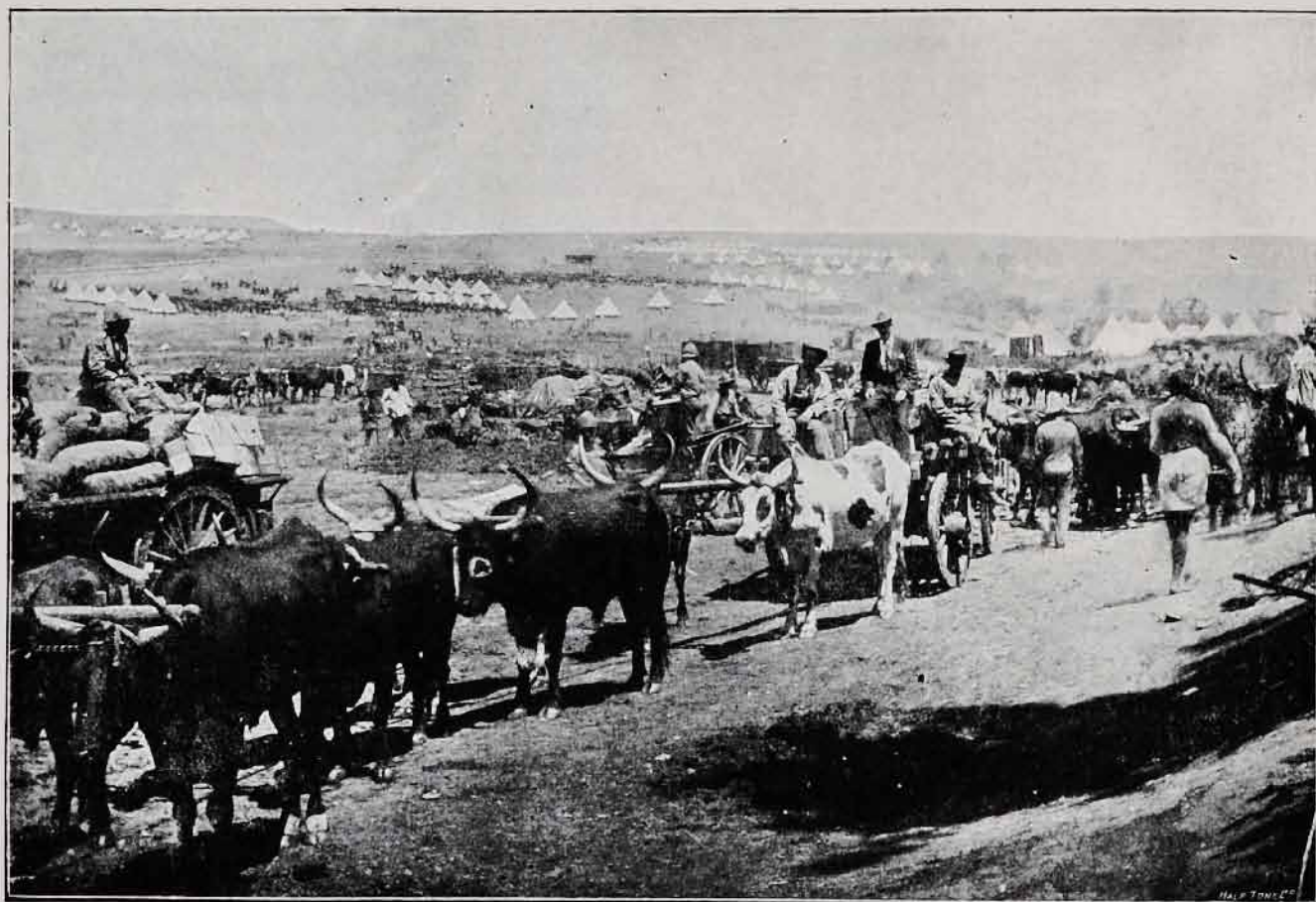
BREAKING CAMP: OX-WAGGONS MOVING OFF.
