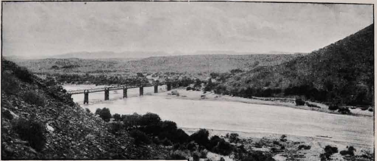
ORANGE RIVER BRIDGE.
