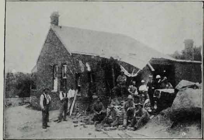
GENERAL WHITE'S HOUSE, LADYSMITH. Damaged by shell fire.
