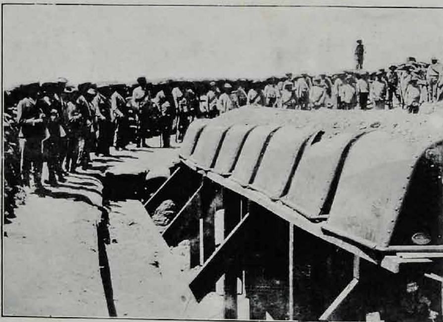
THE SEVENTH AND EIGHTH REDOUBTS AT KIMBERLEY. Partly made of inverted trucks from the mines.
