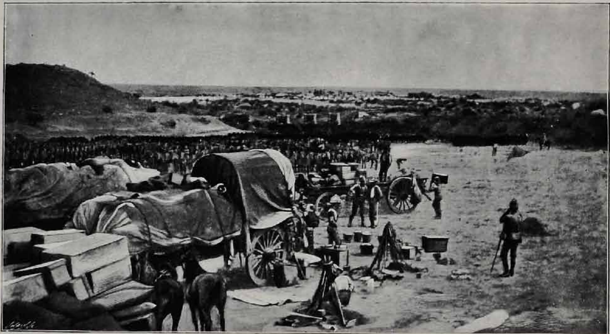
MASSING THE TRANSPORT ON THE NORTH SIDE OF THE TUGELA, OPPOSITE COLENZO. The little town is seen in the centre of the picture just above the piers of the broken bridge.
