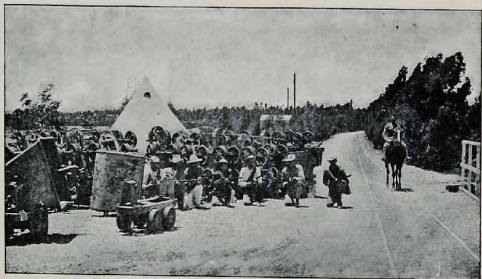
KENILWORTH BARRICADE, FORMED OF THE TRUCKS USED IN THE MINES.
