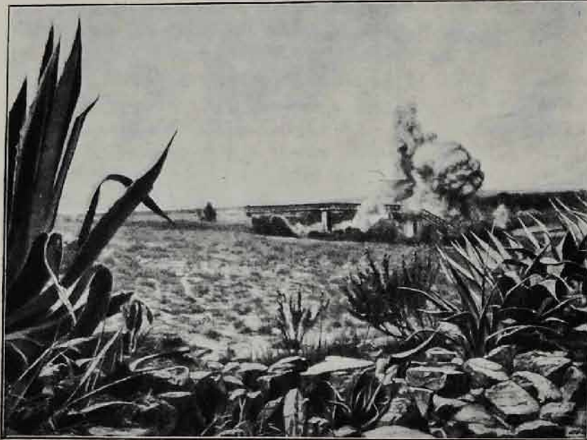
DESTRUCTION OF THE VET RIVER BRIDGE BY THE BOERS.
