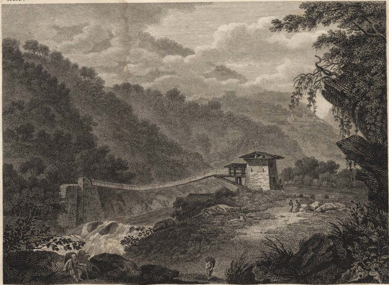
Iron Bridge near Chooka?
