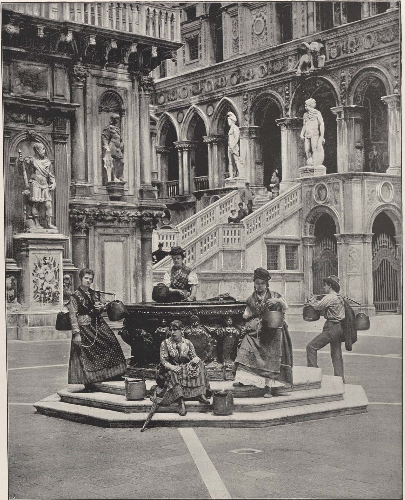
COURTYARD OF THE DUCAL PALACE, VENICE.—In another illustration the exterior of this wonderful building is portrayed, as it fronts upon the Piazzetta. We are here looking on a portion of its inner courtyard, around which rise the marble walls of the Palace, magnificently decorated with stone carving and statuary in bronze and marble. In the foreground is one of two elaborate bronze well-curbs here, the work of Venetian artists 350 years ago. Upon their marble steps Venetian women often sit to rest themselves before returning homeward with their pails of water, gossiping gaily of to-day, unmindful of the history with which each stone in this old building seems at times so eloquent. In the distance we perceive the marble steps, known as the "Giants' Staircase," because of the colossal statues of Mars and Neptune which decorate its summit. This is more than 400 years old, and for centuries at the head of its steps the Doges of Venice were crowned. Byron in his tragedy of "Marino Faliero" makes this the place of that sovereign's execution, and the concluding line of his drama is, "The gory head rolls down the Giants' Steps." Unfortunately, Marino Faliero was decapitated before this stairway had been built, but it is a fact that he was beheaded in this palace. Just beyond the "Giants' Steps" is a flight of stairs leading to the upper story, called the Scala d'Oro, or the Golden Staircase, from the magnificence of its ornamentation.
