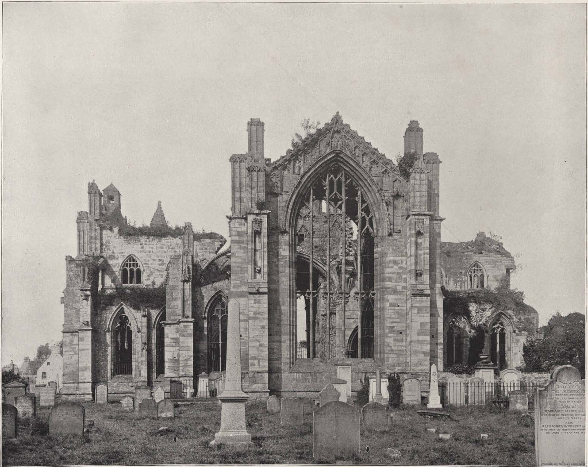
MELROSE ABBEY, SCOTLAND.—The charm of this celebrated structure is proverbial and it well deserves its reputation. Its noble columns, windows and arches are of exquisite beauty and delicate carving, and justify this poetical yet accurate description of Sir Walter: "Thou wouldst have thought some fairy's hand, Twixt poplars straight, an osier wand, in many a freakish knot had twined; Then framed a spell when the work was done, And changed the willow wreaths to stone." This magnificent Abbey was built by King David I, in the twelfth century, and many of the monarchs of Scotland were buried here. Here is also deposited the heart of Robert Bruce. So durable is the red sandstone in which they are chiseled that the most delicately-sculptured capitals and flowers are still perfect, save where the hand of man has injured them. Yes, the "hand of man," for the mere lapse of time would not have caused such overthrow as this. Alas! it has been almost universally the fact that man himself has shattered the most exquisite and wonderful structures which human genius has been able to create. So was it here. Again and again contending armies plundered it, and finally the Scotch Reformers did even more injury to its remaining statues and carving than had been effected by the ravages of war! The sight of this ruined pile at moonlight can never be forgotten and imparts forevermore a new charm to the well-known lines of Scott: "If thou wouldst view fair Melrose aright, Go visit it by the pale moonlight, When buttress and buttress alternately Seemed framed of ebony and ivory; And home returning, soothly swear, Was never scene so sad and fair."
