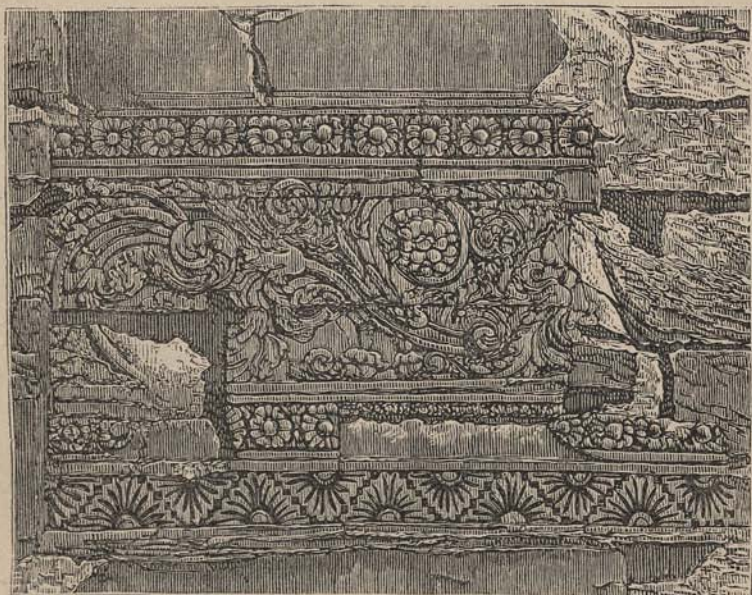
CARVING ON THE TOWER AT SARNATH.
