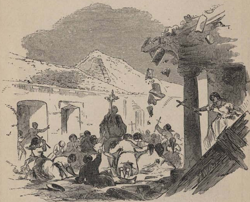
STREET SCENE DURING AN EARTHQUAKE.
