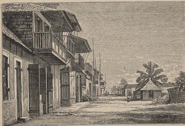
A STREET IN POINT DE GALLE.
