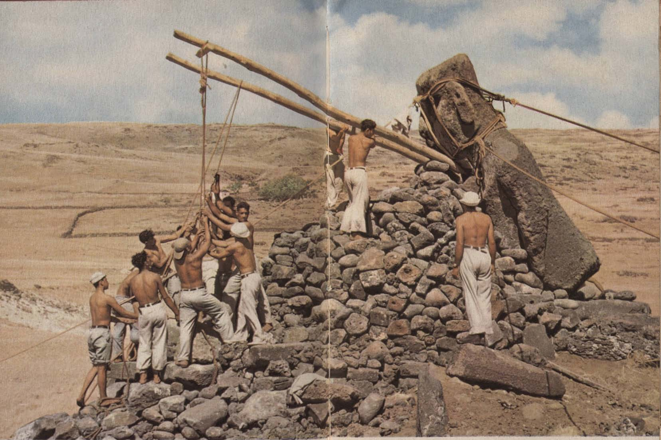
With a heap of stones under its stomach the figure moves upwards and backwards until it stands in its old place on the wall. Twelve men with poles and stones set it up in eighteen days. On the last day the giant is held by ropes to prevent it from toppling off the high wall when it is tilted into the standing position.
