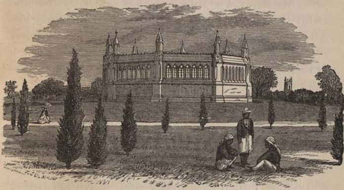
MEMORIAL WELL, WITH CHURCH IN DISTANCE.
