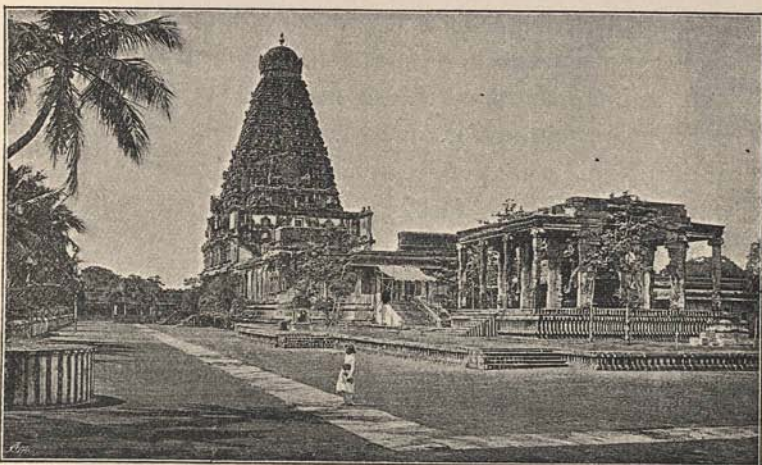
TEMPLE AT TANJORE, GENERAL VIEW.
