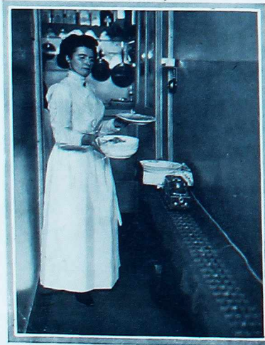
The Kitchen to Dining-room Electric Railway The cook loading the train with salad
