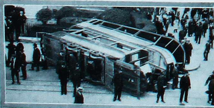
AN ELECTRIC CAR ACCIDENT.
