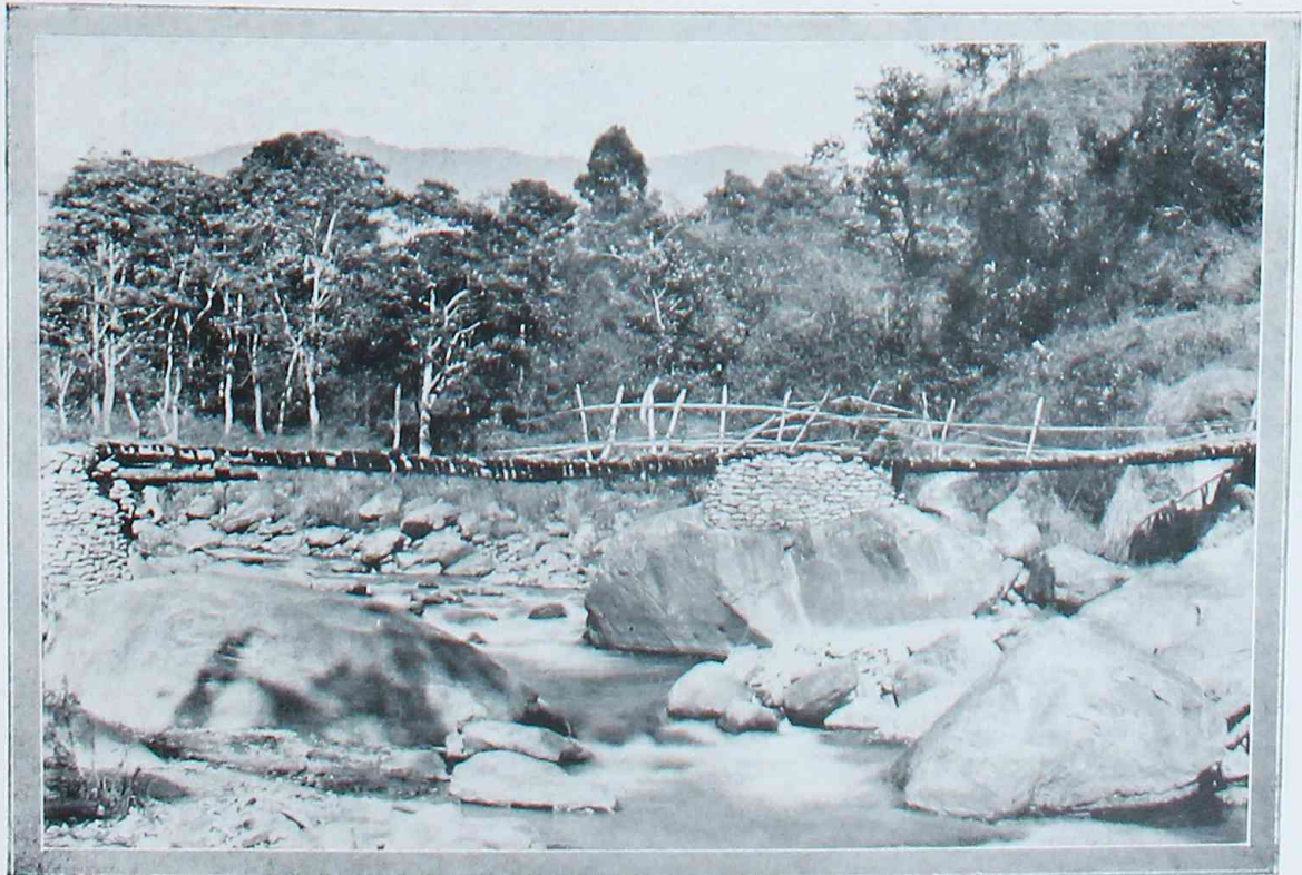
Rustic Cantilever Bridge in the Darjeeling District.
