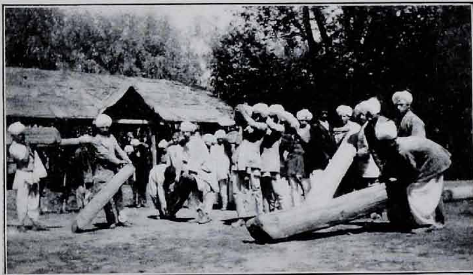
ISLAMABAD BOYS CARRYING MATERIALS FOR CONSTRUCTING NEW SCHOOL BUILDINGS
