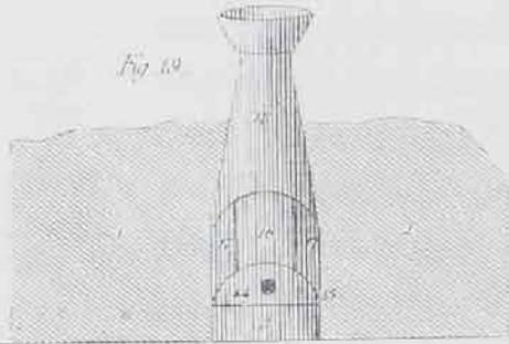
Longitudinal section of the tamping furnace.
