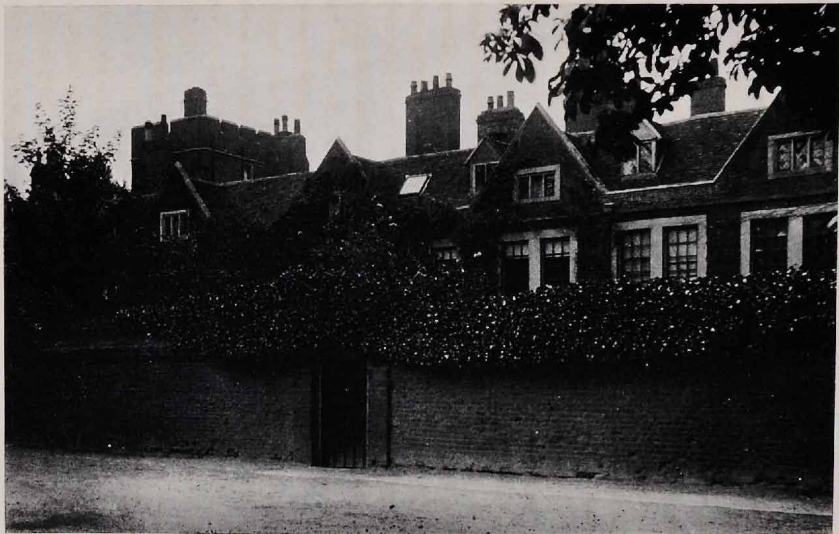
HOUSE IN WESTON'S YARD BUILT IN 1603-6 FOR SIR HENRY SAVILE'S PRINTING PRESS.
