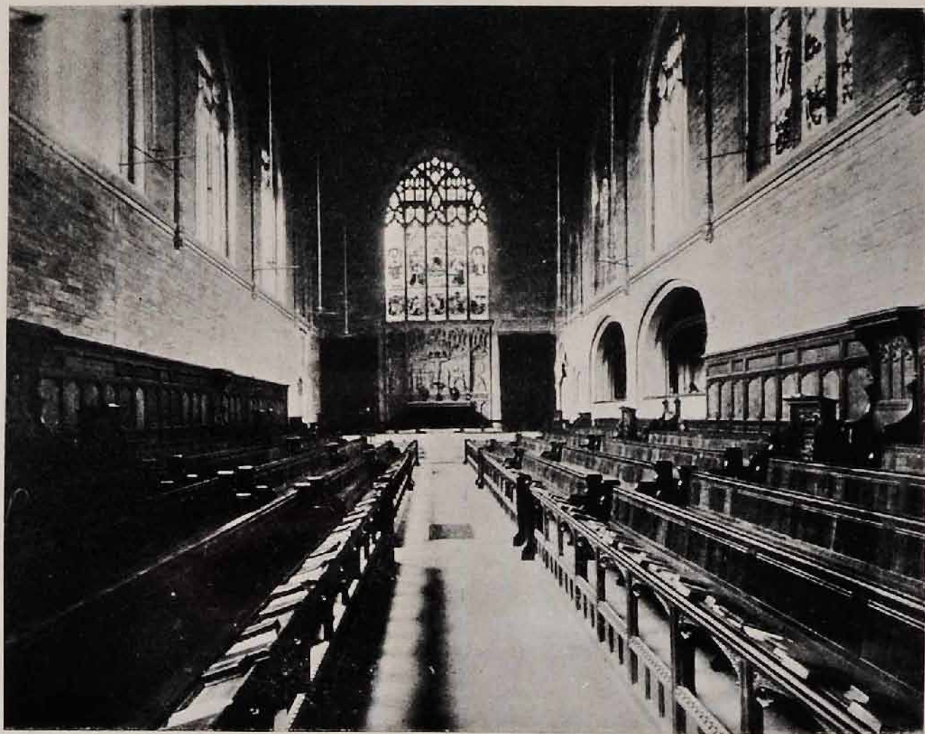
LOWER CHAPEL LOOKING EAST
