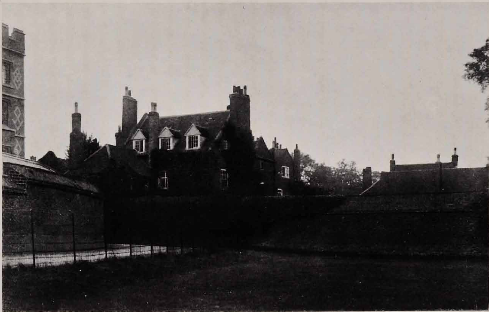
HOUSE BY THE PLAYING FIELDS' ENTRANCE FORMERLY HEXTER'S WHERE SHELLEY BOARDED.
