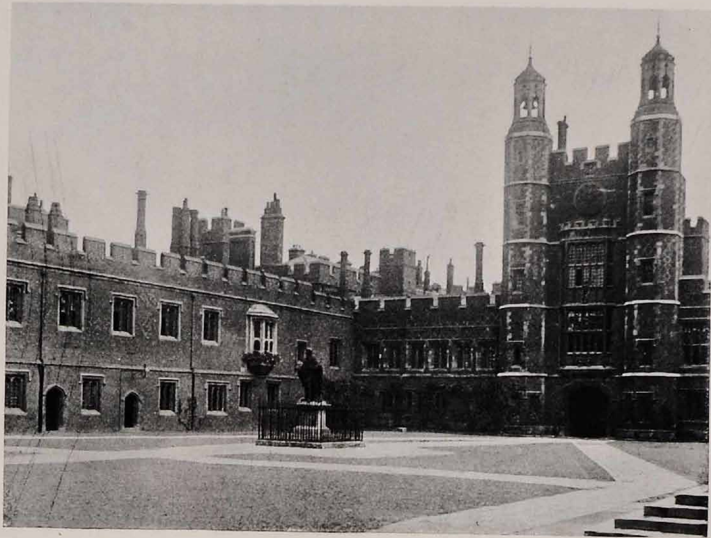
SCHOOL YARD WITH PART OF LONG CHAMBER AND LUPTON'S TOWER
