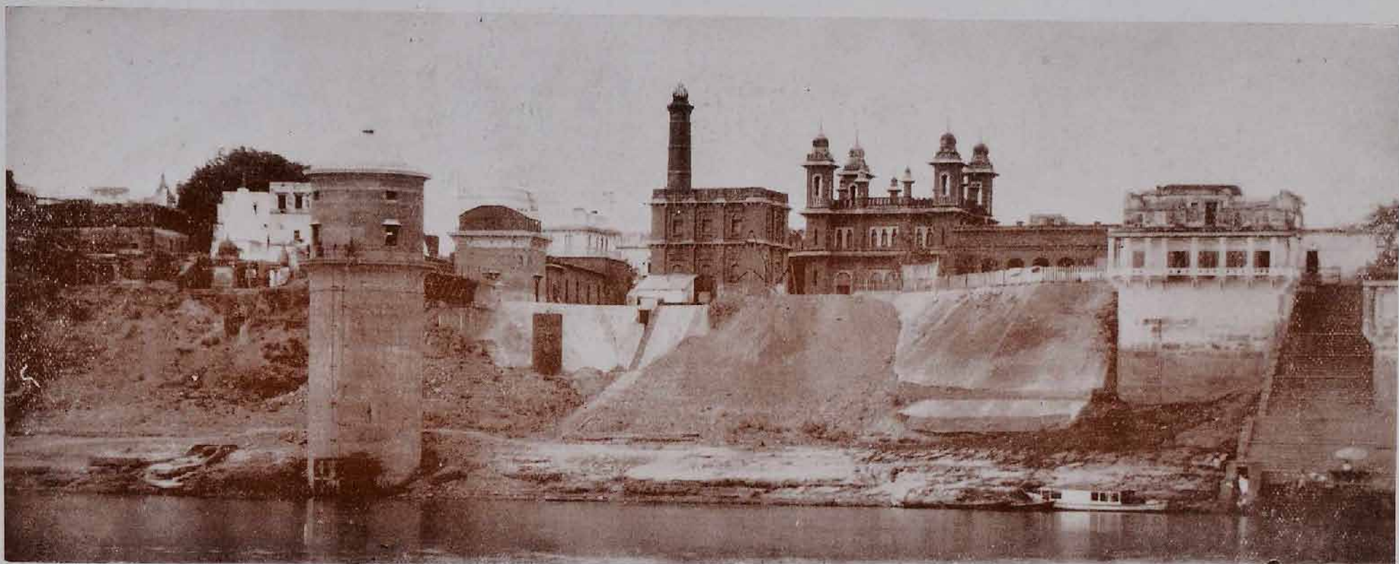
Bhadaini Water Works
