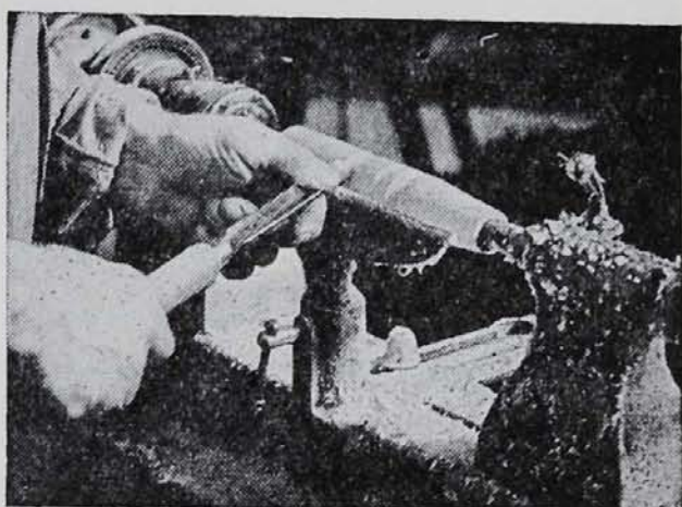
FIG. 2.143. Cutting away waste stock with a gouge.
