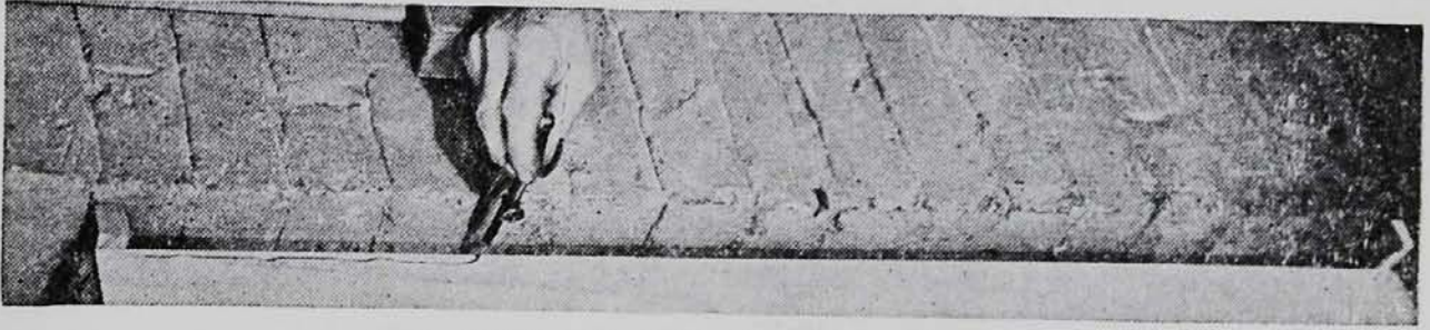
FIG. 2.134. Scribing line for scribed joint.
