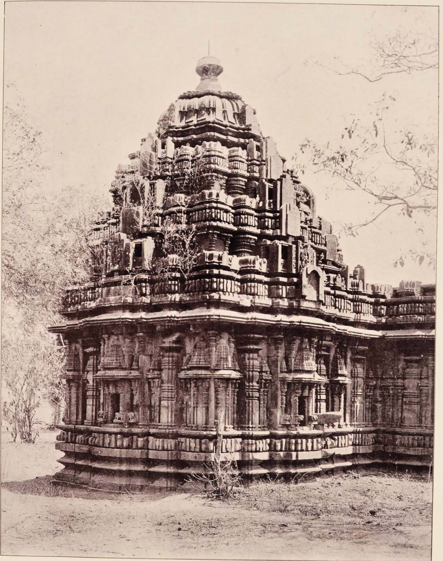
TILIVALLI: SHRINE WALLS AND TOWER OF SANTESVARA.
