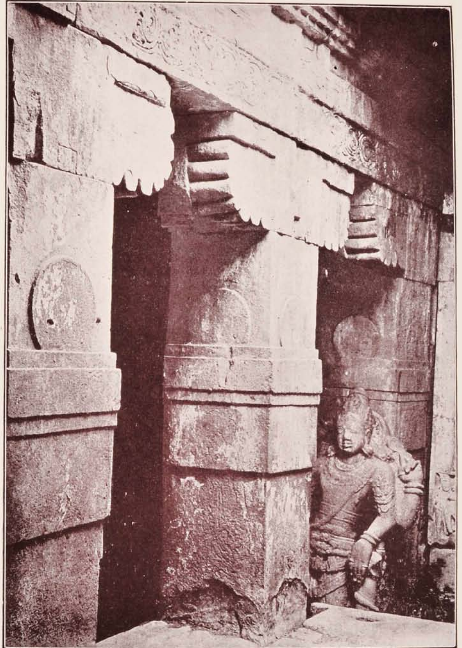
AIHOLE: PILLARS IN TEMPLE NO. 10.
