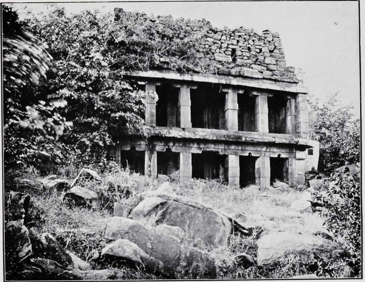
Fig. 6.—The two-storeyed Jaina temple, Aihole.
