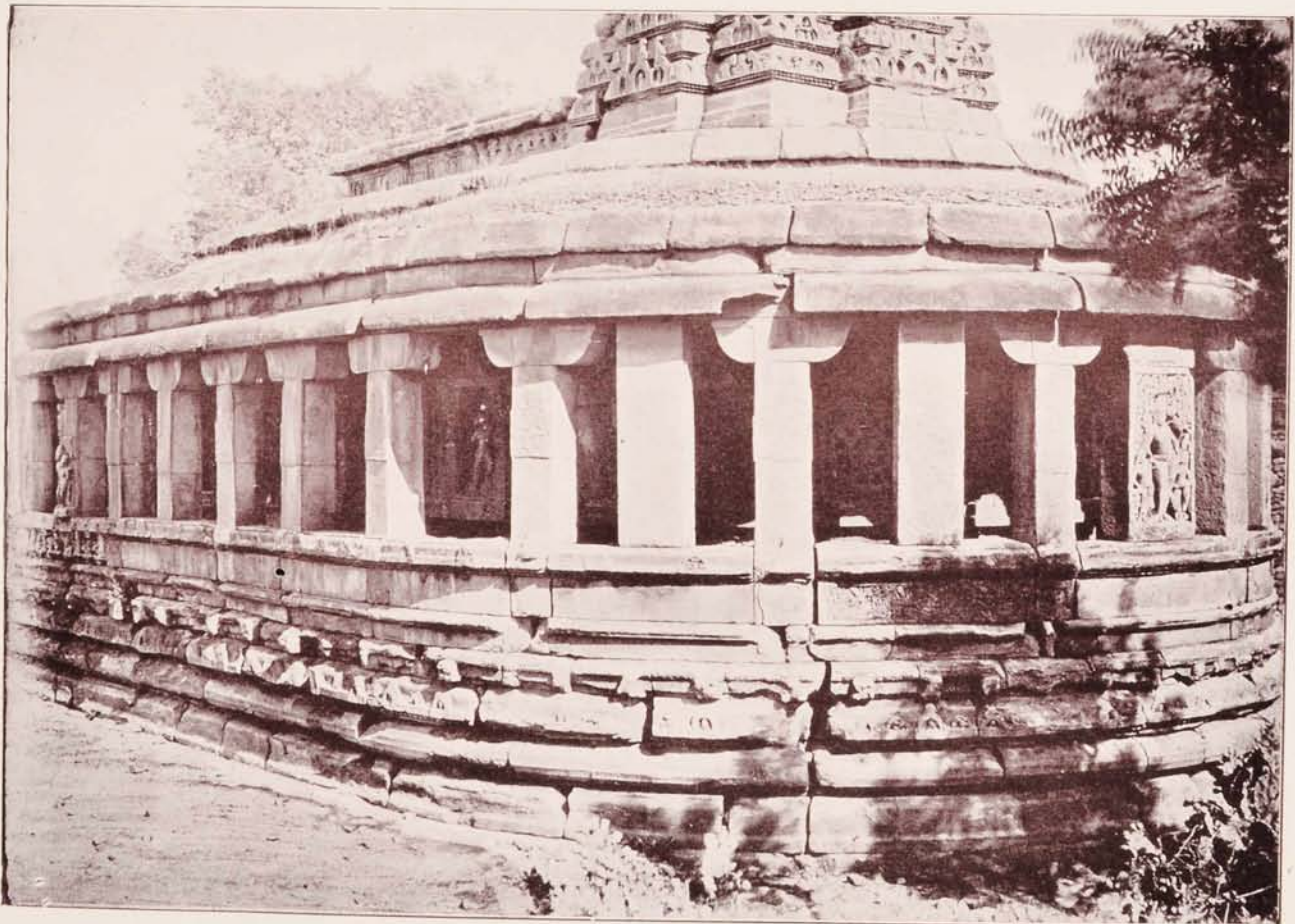
AIHOLE: THE DURGA TEMPLE FROM THE NORTH-WEST.
