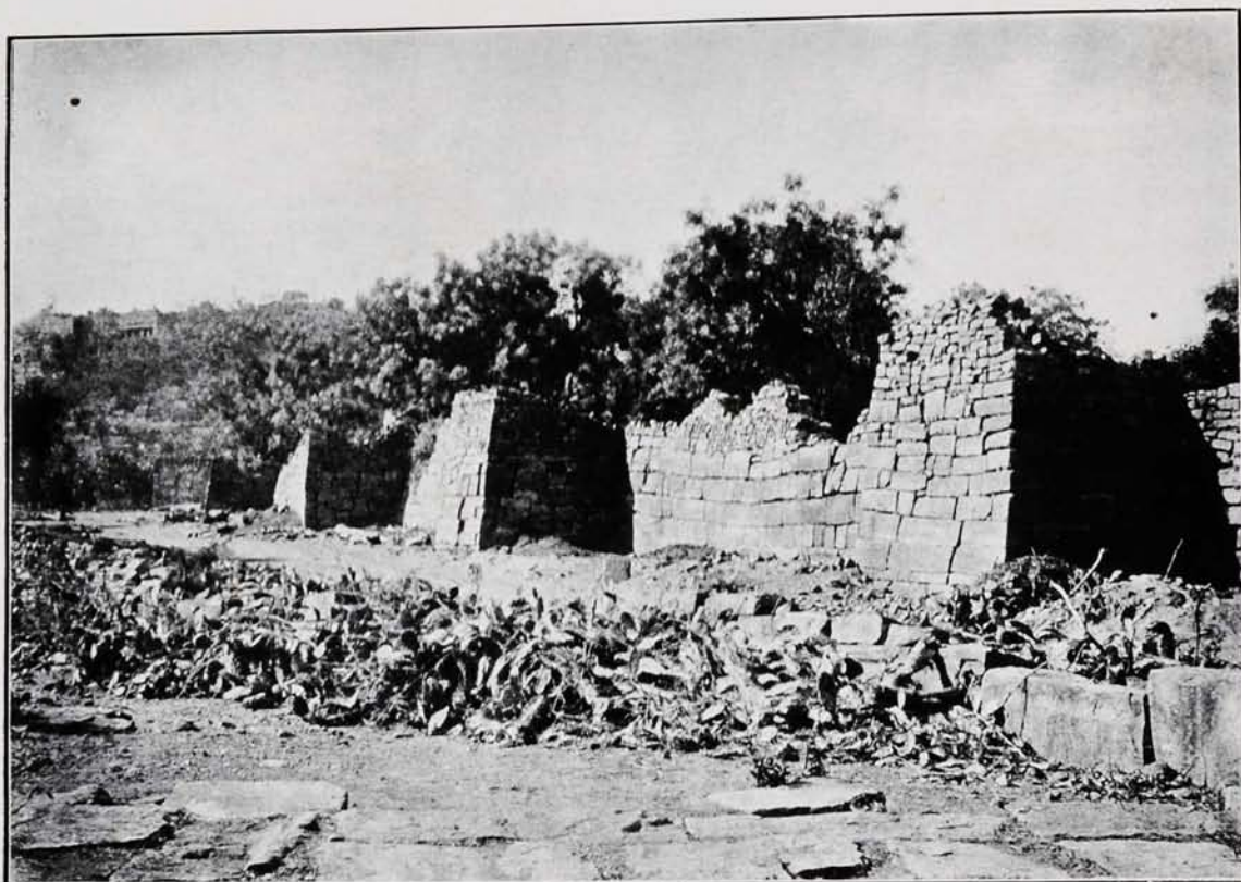
Fig. 4.—The old walls of the village of Aiḥole.
