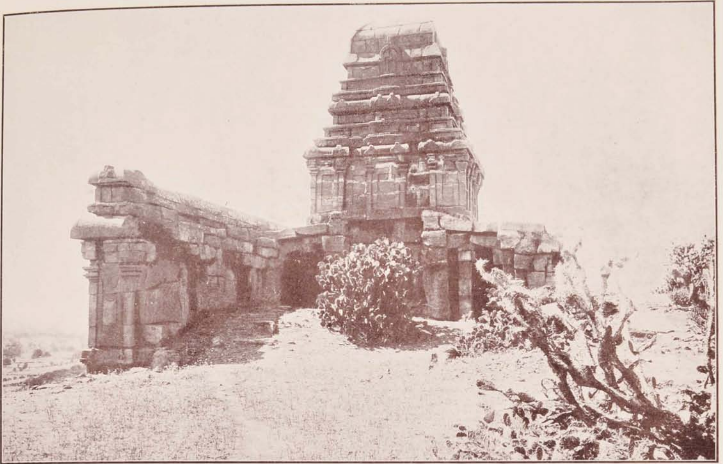
BADAMI: RUINED TEMPLE ON THE NORTHERN FORT FROM THE EAST.
