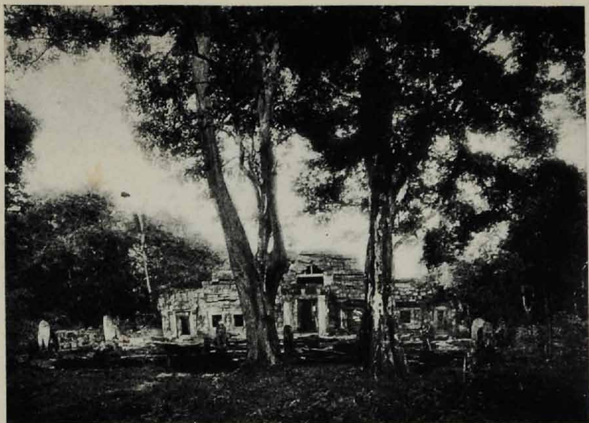
BANTEI KEDEI Eastern portal of the inner wall
