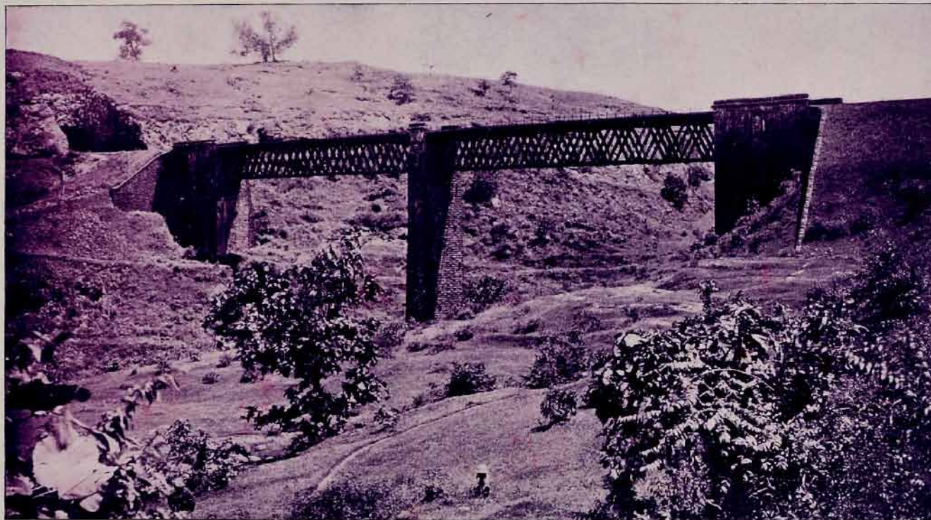
VIADUCT ON THE GHÂTS, G. I. P. RAILWAY.
