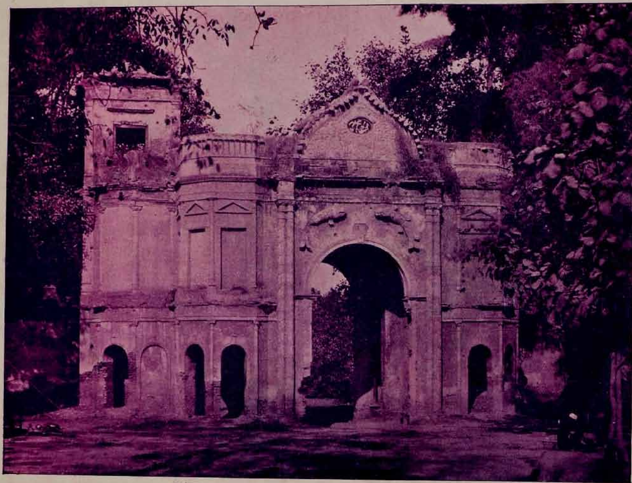
ENTRANCE GATE, SECUNDRABAGH, LUCKNOW.
