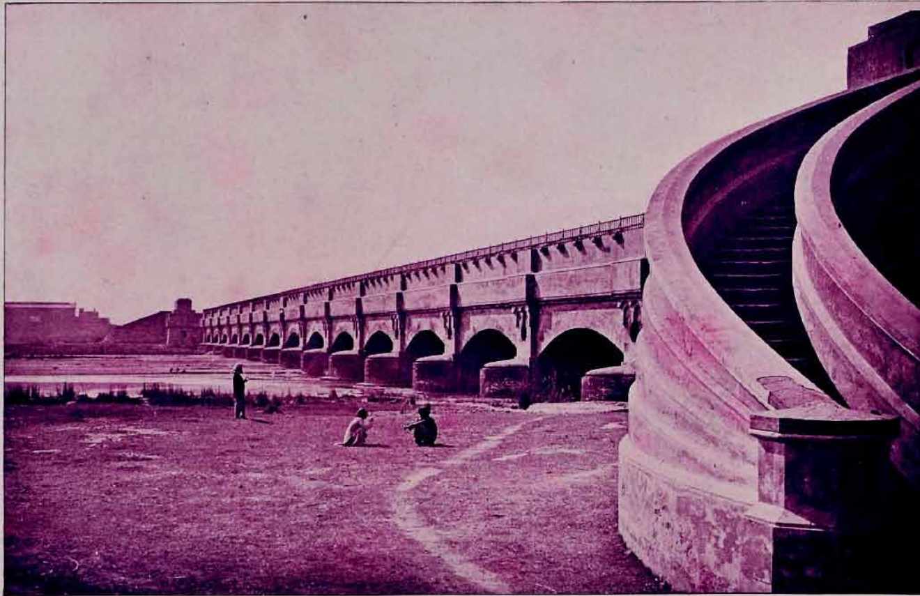
AQUEDUCT OF THE GANGES CANAL, ROORKEE.
