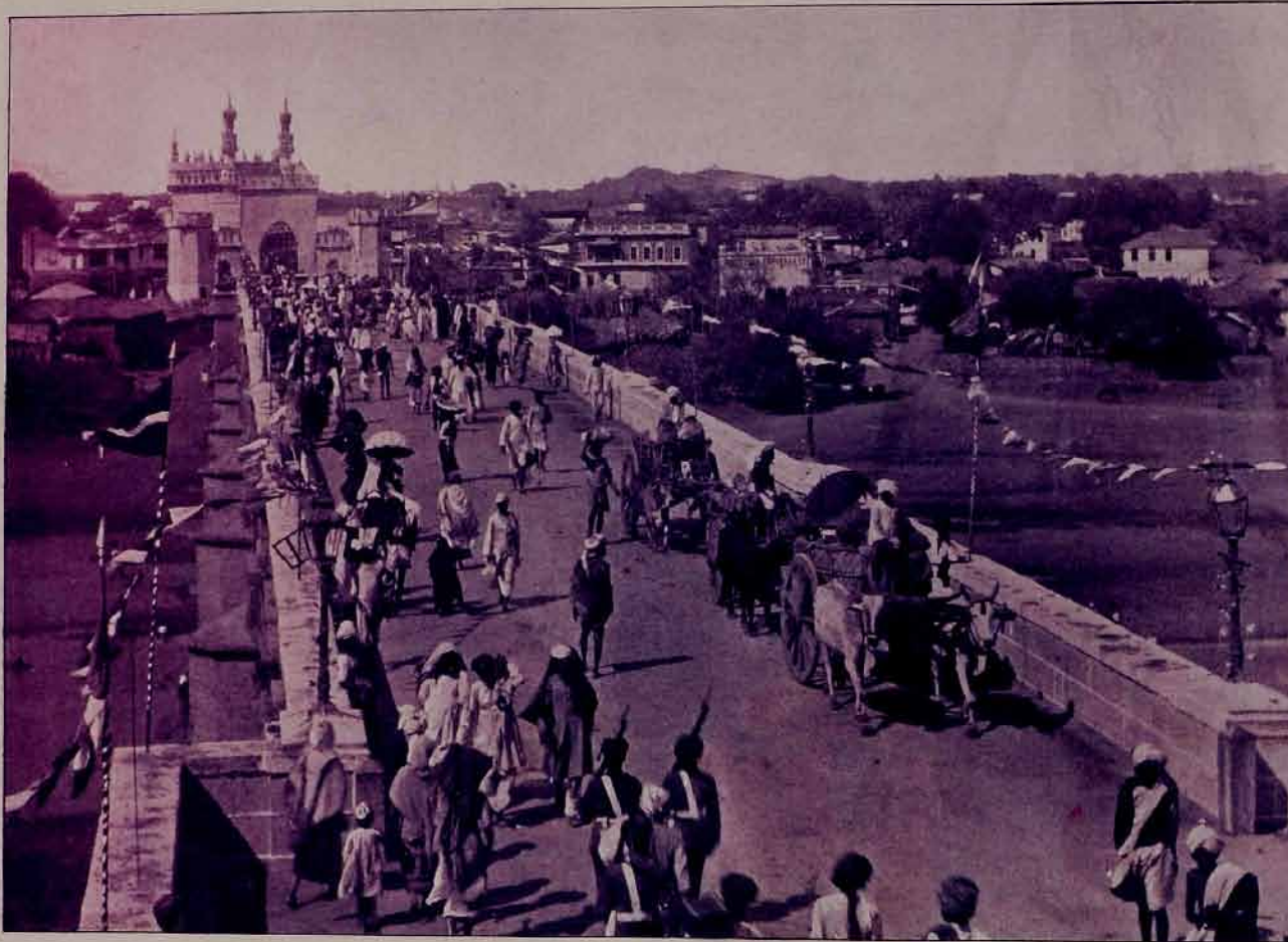
THE AFZAL BRIDGE, HYDERABAD.
