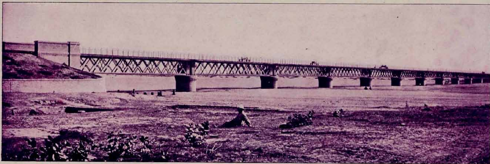
RAILWAY BRIDGE NEAR UMBALLA.
