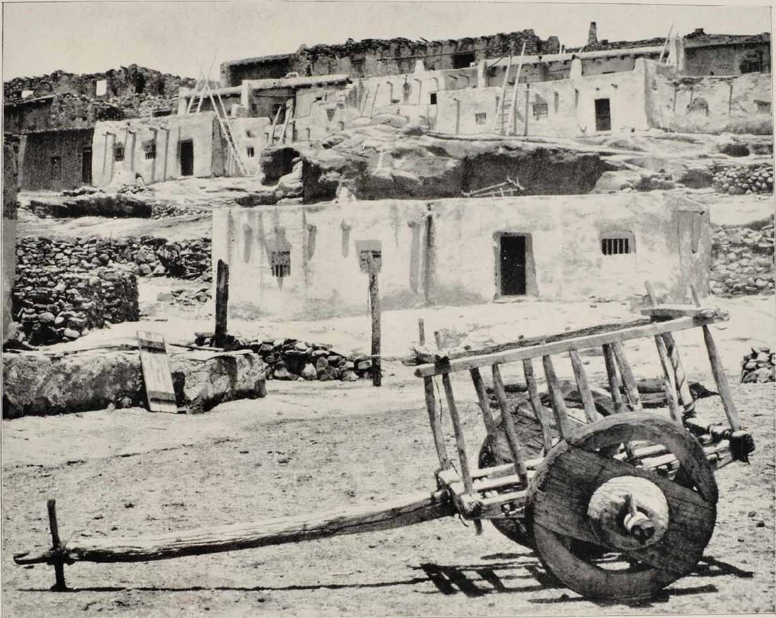
ADOBE HOUSES, NEW MEXICO. —In "New" Mexico and in "Old" Mexico there is a peculiar style of architecture which is both primitive, natural and economical—it is the ADOBE method of building. Large flat cakes of sun-dried clay, called "Adobe bricks," are used to-day and have been used for ages in these countries. In fact, we find the same thing to have been done in Egypt and the Holy Land, and many a town in Mexico presents a decidedly Oriental appearance on account of its thousands of flat-roofed houses of adobe. It can not be said of this material that it is at all beautiful. The color of such houses is far from cheerful, being frequently a sort of compromise between a loaf of brown-bread and a strong cigar. There are rarely any windows in these huts and almost never does a chimney rob them of their flatness and monotony. But as a rule in New Mexico, as in the country south of the Rio Grande, no fires are needed either for warmth or cooking, save such as can be made in a pan, or at best, in small brick ovens, heated with charcoal. One-half the world, it is said, does not know how the other half lives. To see these dwellers in adobe huts is quite a revelation to most travelers; but who knows whether their inhabitants are not in reality as happy as the wealthy inmates of a sumptuous palace?
