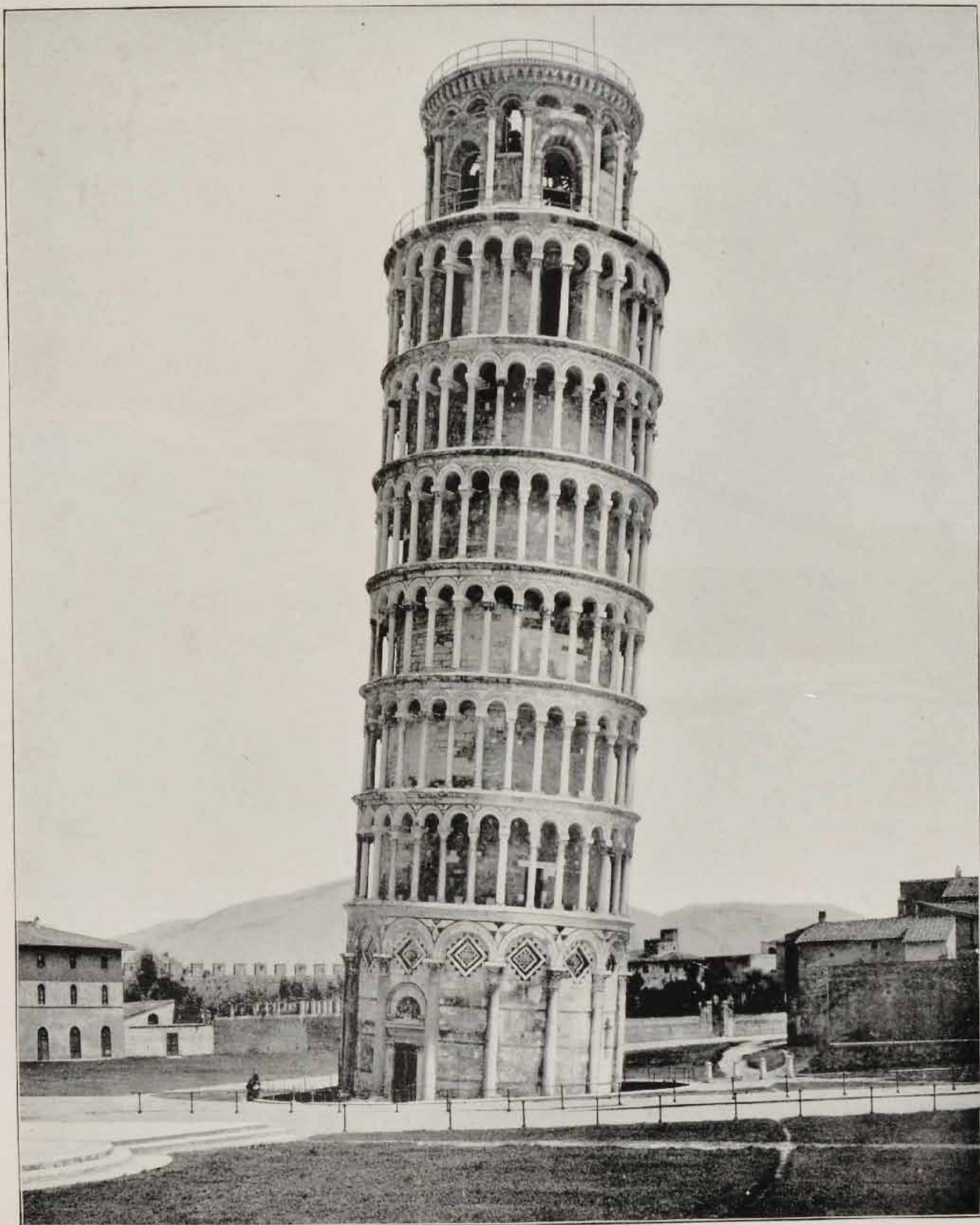
LEANING TOWER, PISA.—The city of Pisa is known throughout the world from the fact that it possesses a structure which is so far inclined from the perpendicular as to appear to be on the point of falling. Moreover, this leaning tower is as beautiful as it is extraordinary. It is of pure white marble, and the delicate colonnades which encircle it, ascending in a spiral to the lofty belfry, are marvels of grace and elegance. It has a height of about 180 feet, and is fourteen feet out of perpendicular. It is hollow inside, and looking from the top down its cylindrical interior is like gazing into a well. In spite of one's conviction that a tower which has been leaning thus for nearly 600 years will not fall, it is impossible to avoid a slight feeling of nervousness, as one looks down from the lower side of the upper gallery. The sensation is peculiar, and one clutches the iron railing as he surveys beneath him the retreating marble wall. Close by this tower are other buildings which would make Pisa famous even without the assistance of its "leaning miracle," namely, its grand cathedral of white marble, where there still hangs the chandelier whose oscillations led Galileo to invent the Pendulum. The Baptistery also is another marble building of remarkable beauty and possessing a marvelous echo, while the Campo Santo or Cemetery of Pisa close at hand, is a cloistered structure adorned with many statues, mediæval monuments and splendid tombs.
