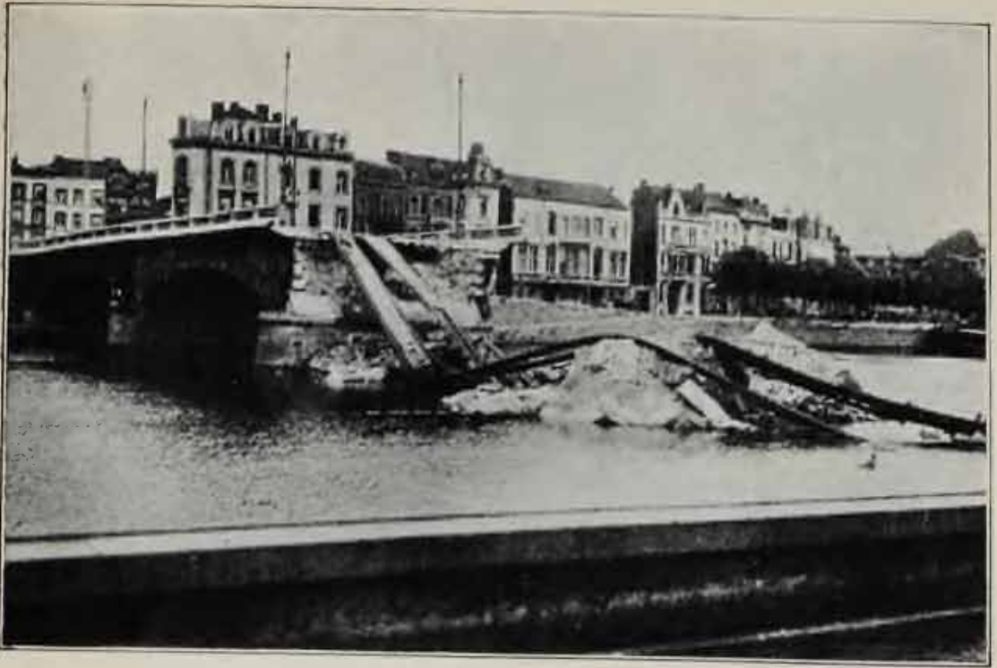
ANOTHER VIEW OF THE RUINED BRIDGE.
