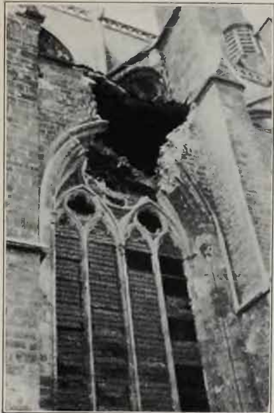
MALINES CATHEDRAL. Window destroyed by German shell. (Underwood & Underwood.)
