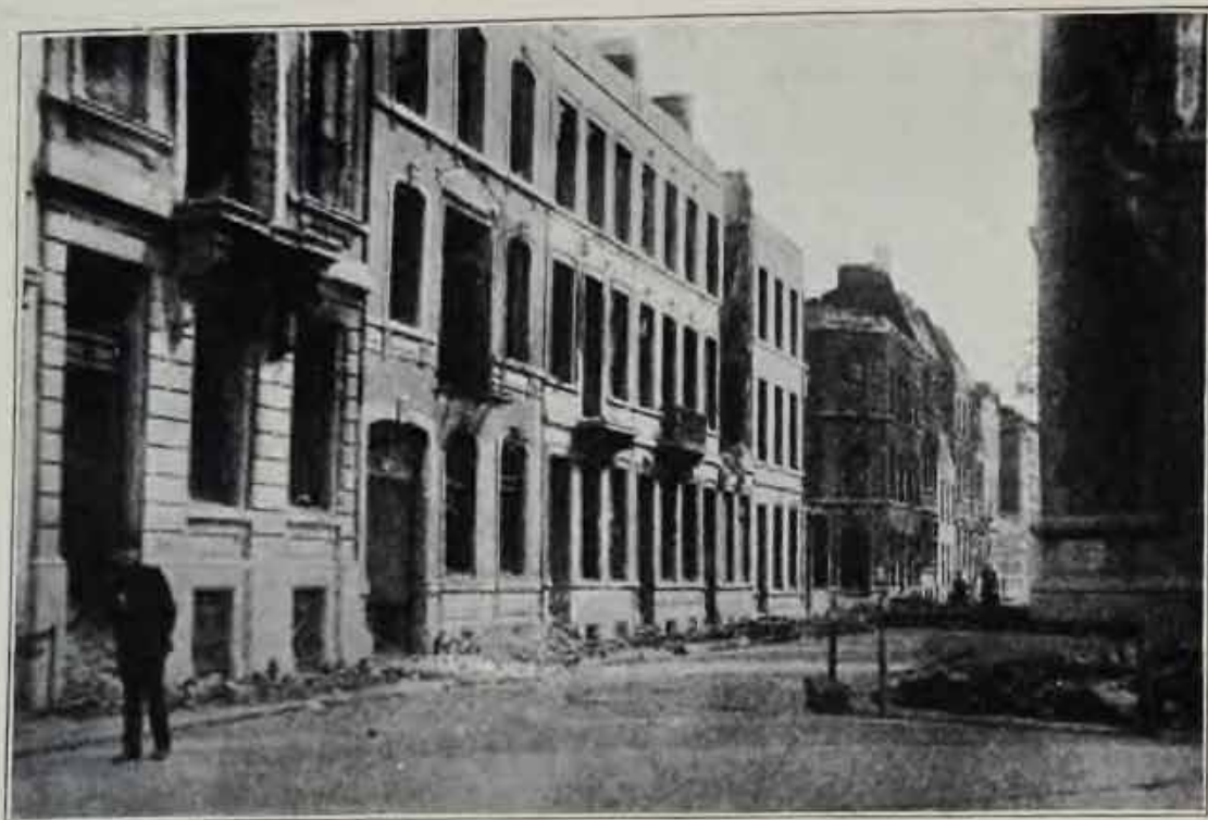
A RUINED STREET IN LIEGE.
