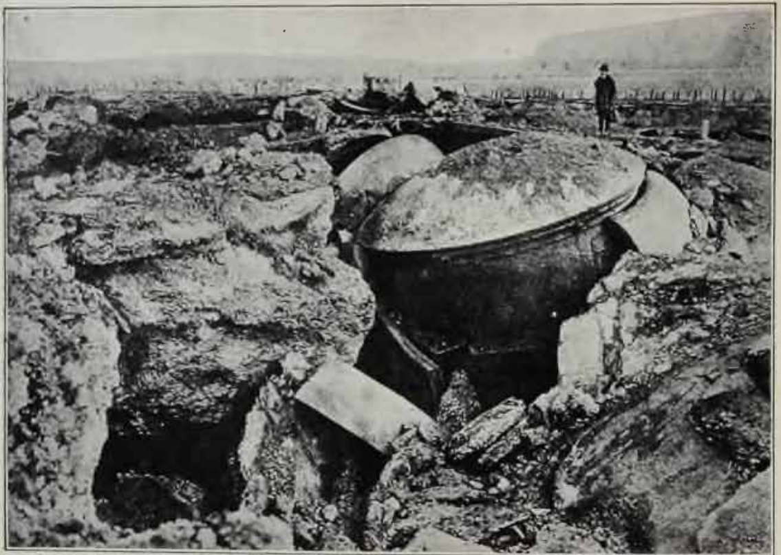
ONE OF THE FORTS AT LIÈGE AFTER BOMBARDMENT. Showing damage caused by German siege guns.
