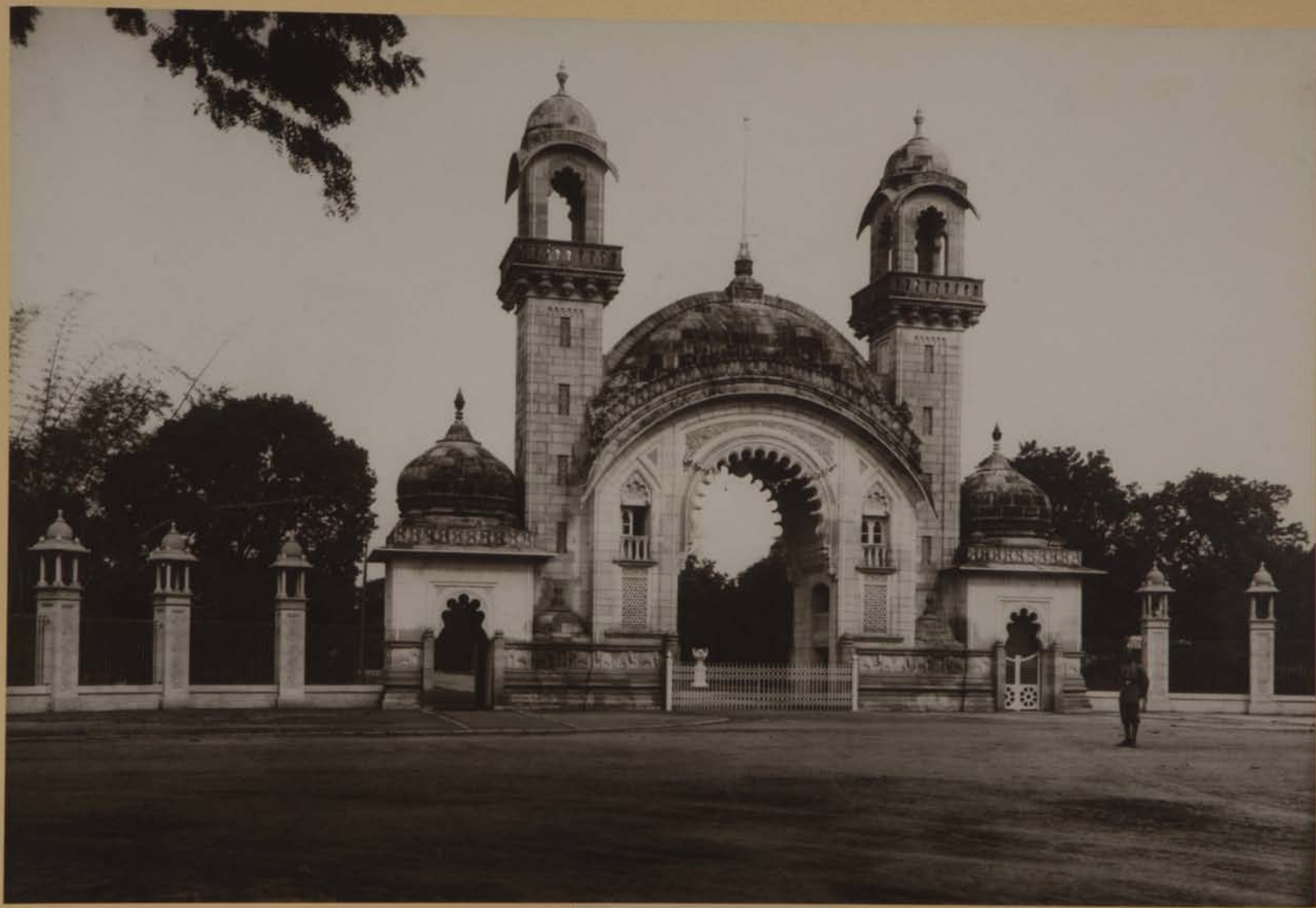
Main Gate Laxmi Vilas Palace.
