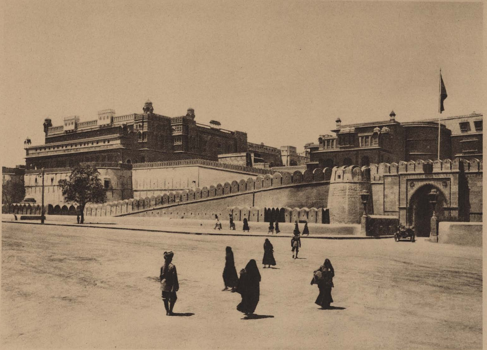
THE FORT GATE
